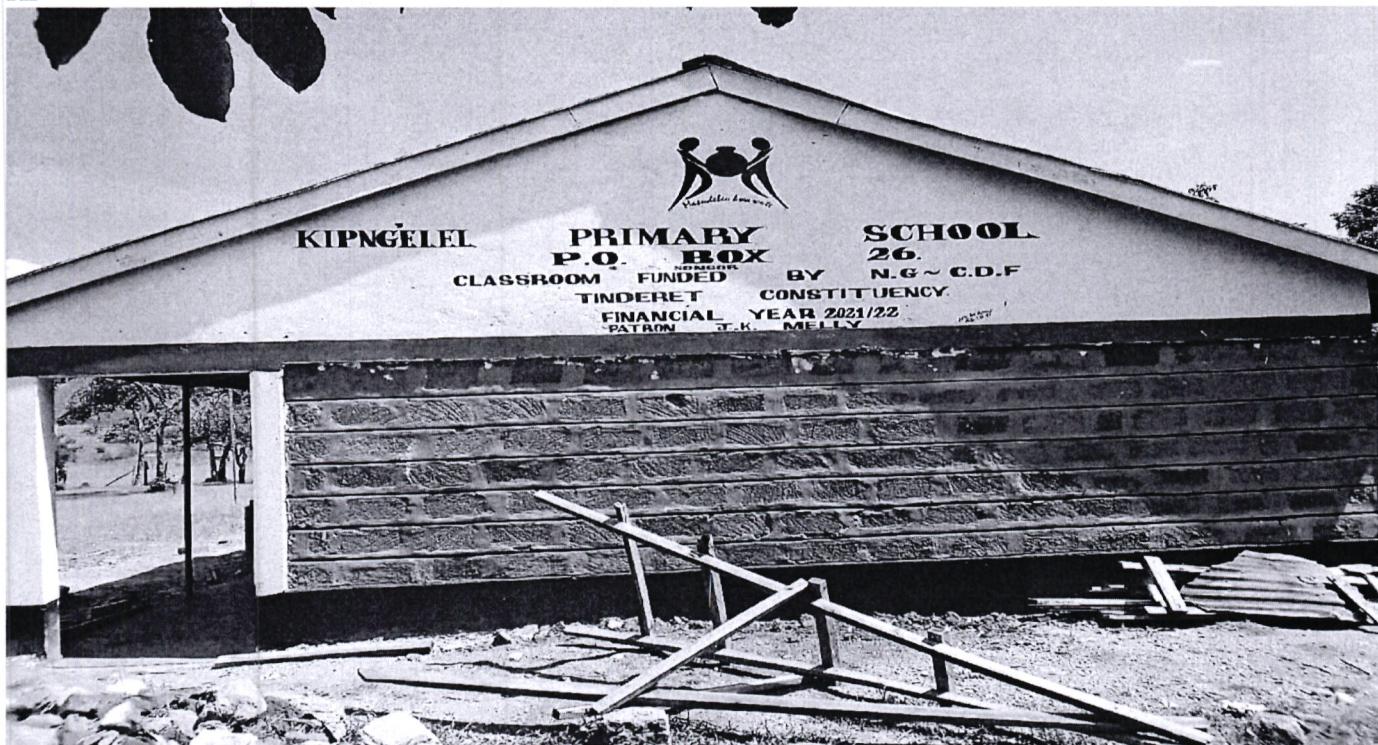
Kipng'elel Primary School: Construction of 1 classroom to completion.
