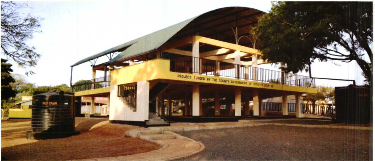
Modern Market Shed at Matinyani - Kitui County
