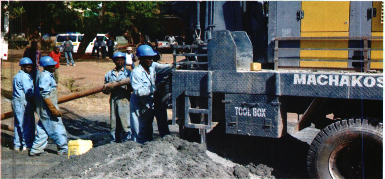
Drilling of a borehole in Machakos County
