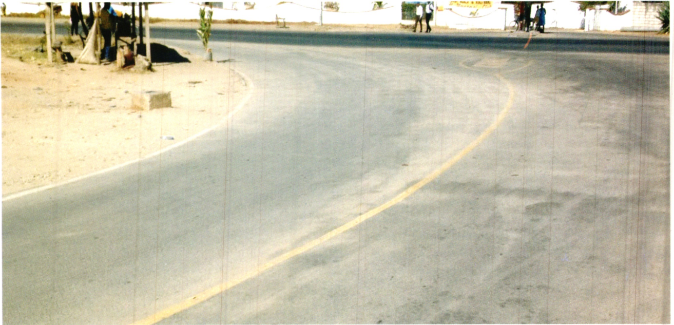
Upgraded bitumen standard road at Junction Mnarani to Old Ferry in Kilifi County.
