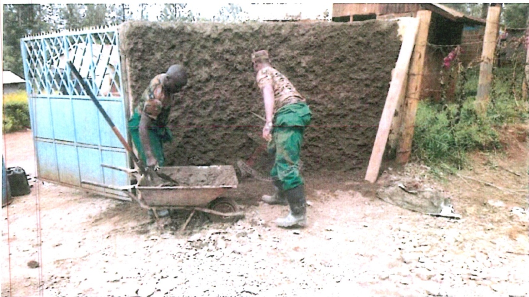
Rehabilitation of Witathani School
