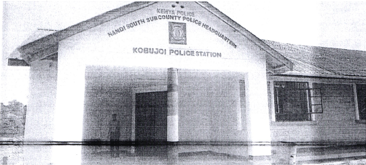
Kobujoi Police station construction of the station
