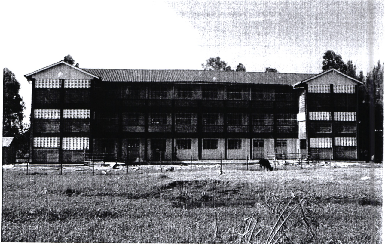
Fig. 3: Construction of 12 no classrooms at Dago primary school.
