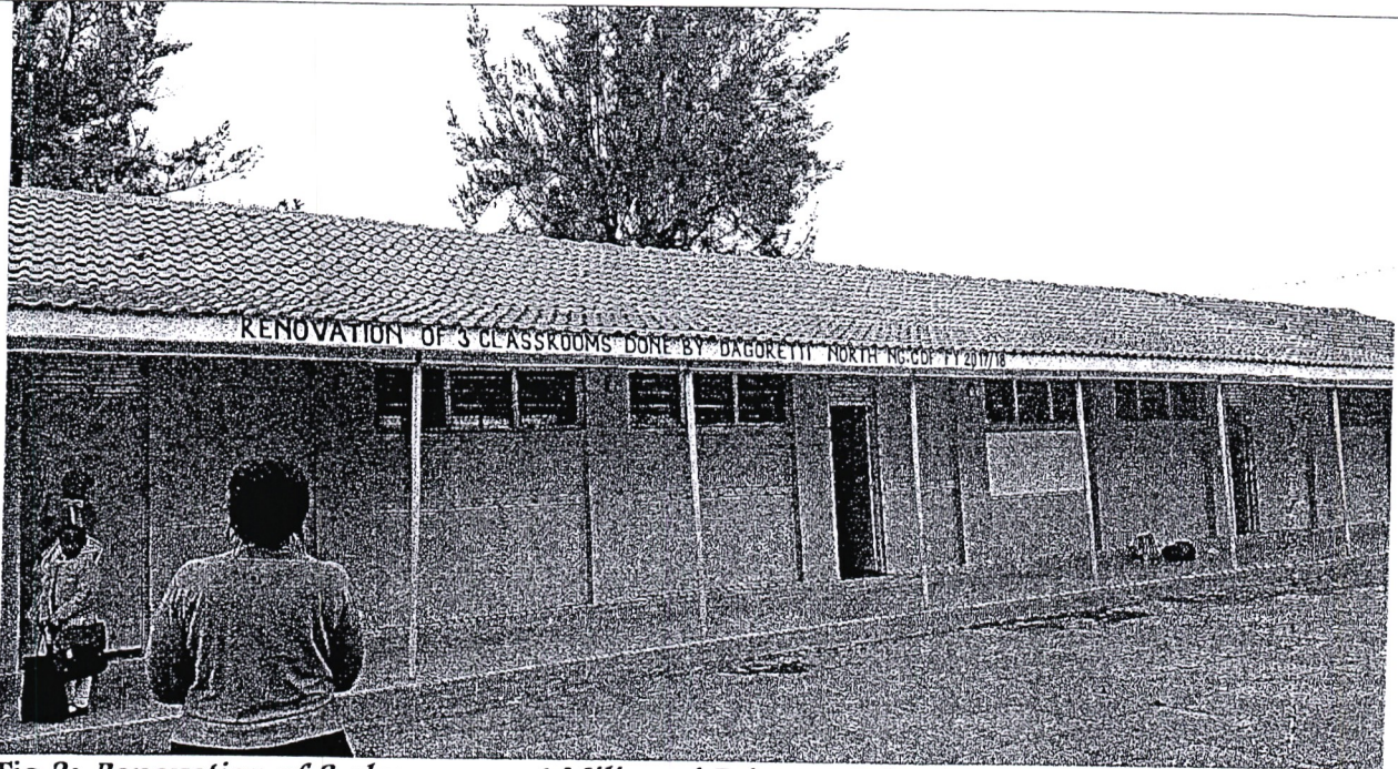
Fig 2: Renovation of 3 classrooms at Milimani Primary School.
