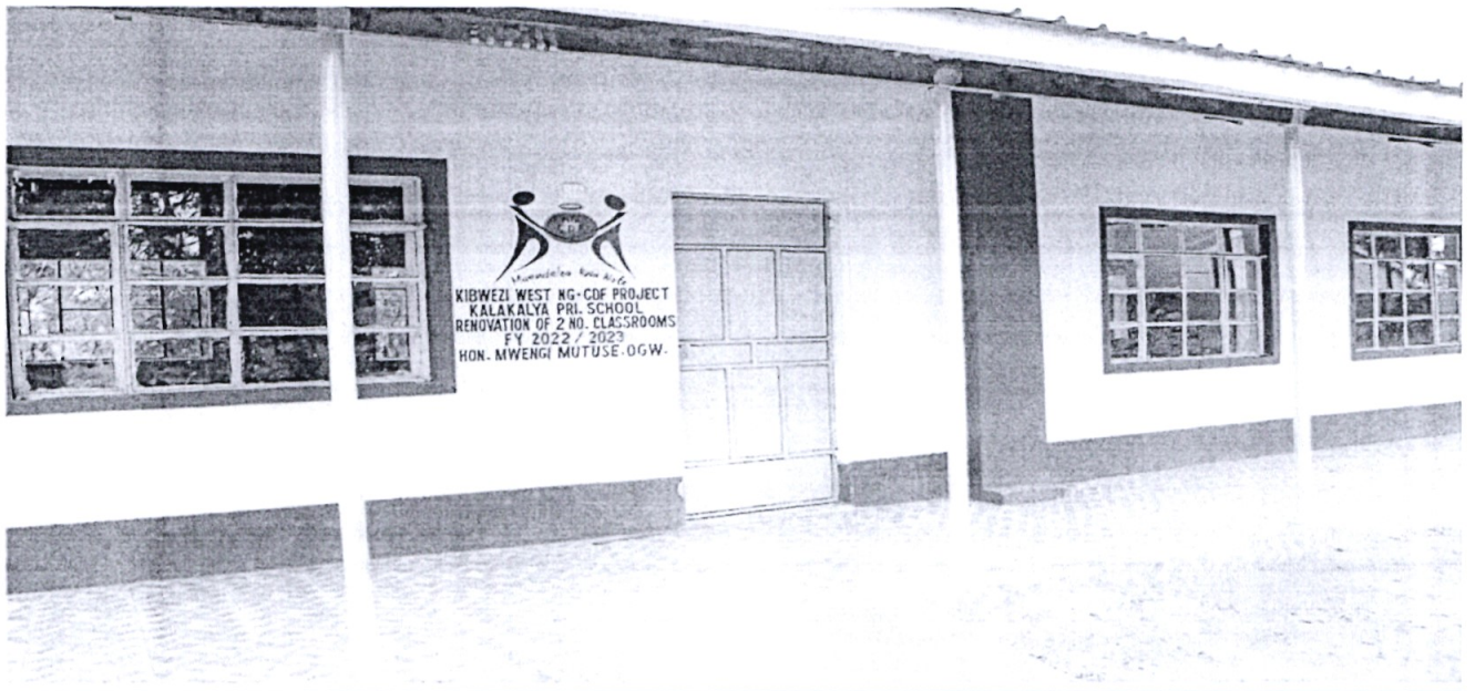
RENOVATION OF 2 NO. CLASSROOM BLOCK AT KALYAKALYA PRIMARY SCHOOL.
