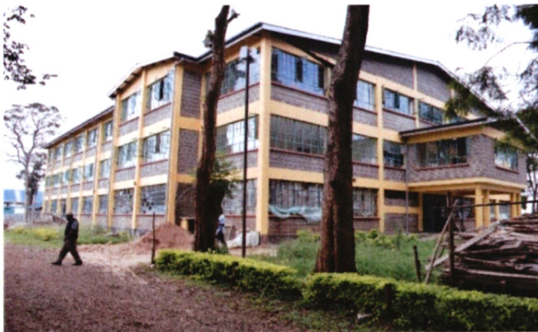
Phase II Construction of Electoral Engineering workshop
