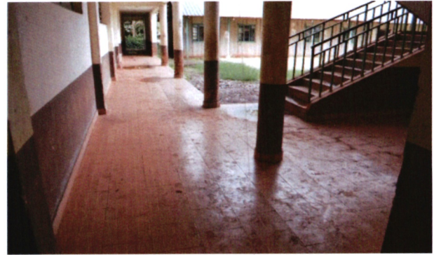
Block K Classroom Floor tiling
