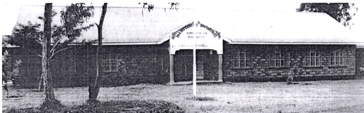
Figure 1: Wang'chieng Divisional Headquarters - Construction of Administration Block to completion
