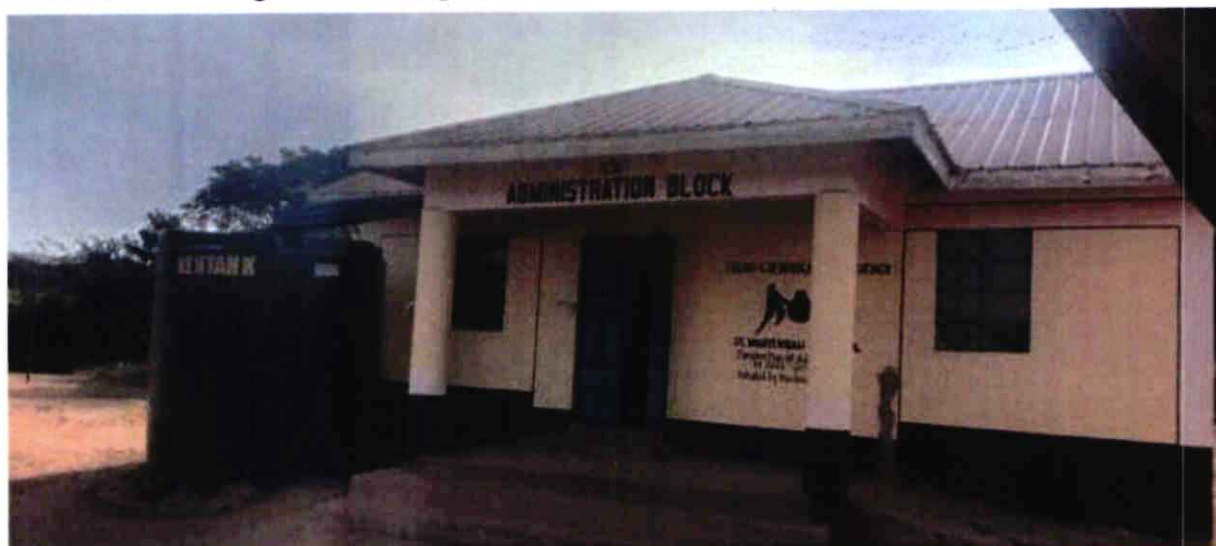
Pic 1.2 St. Marys Kibau Secondary School ; Construction of Administration Block
