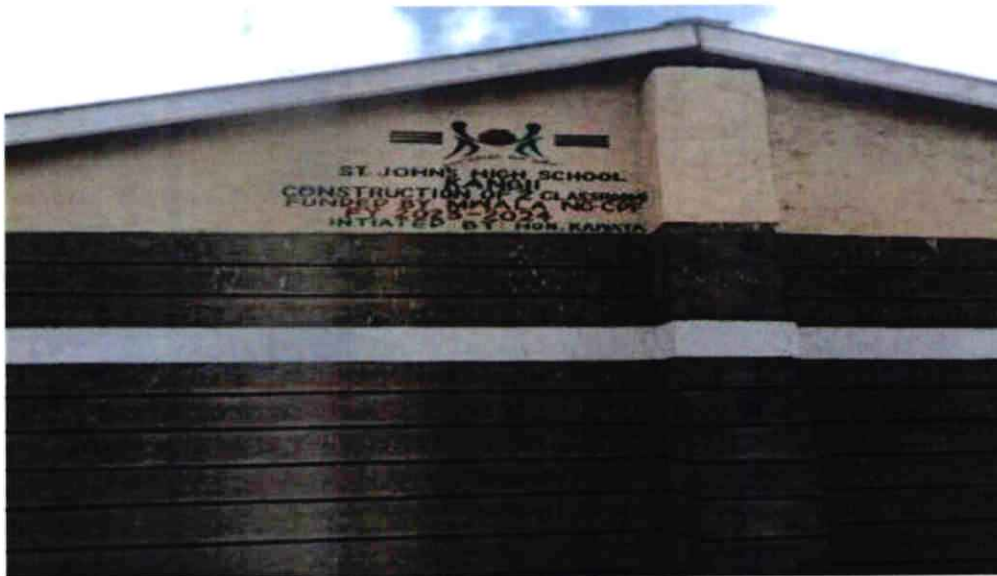
Pic 1.1 St. Johns High School Kangii ; Construction of 2 classrooms
