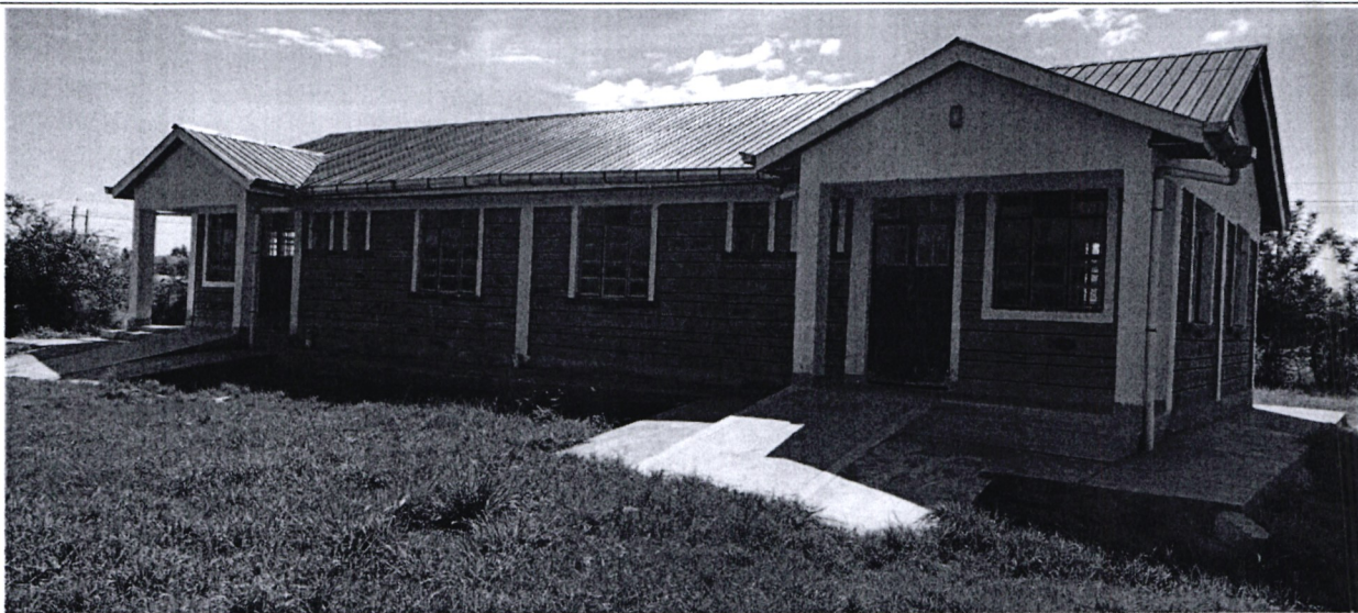
Fig 4: construction of staff quarters at Kibos secondary school.
