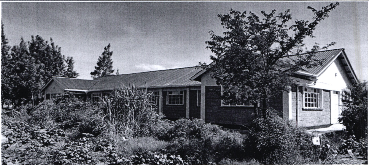
Fig 2: construction of a dormitory at kibos secondary school.
