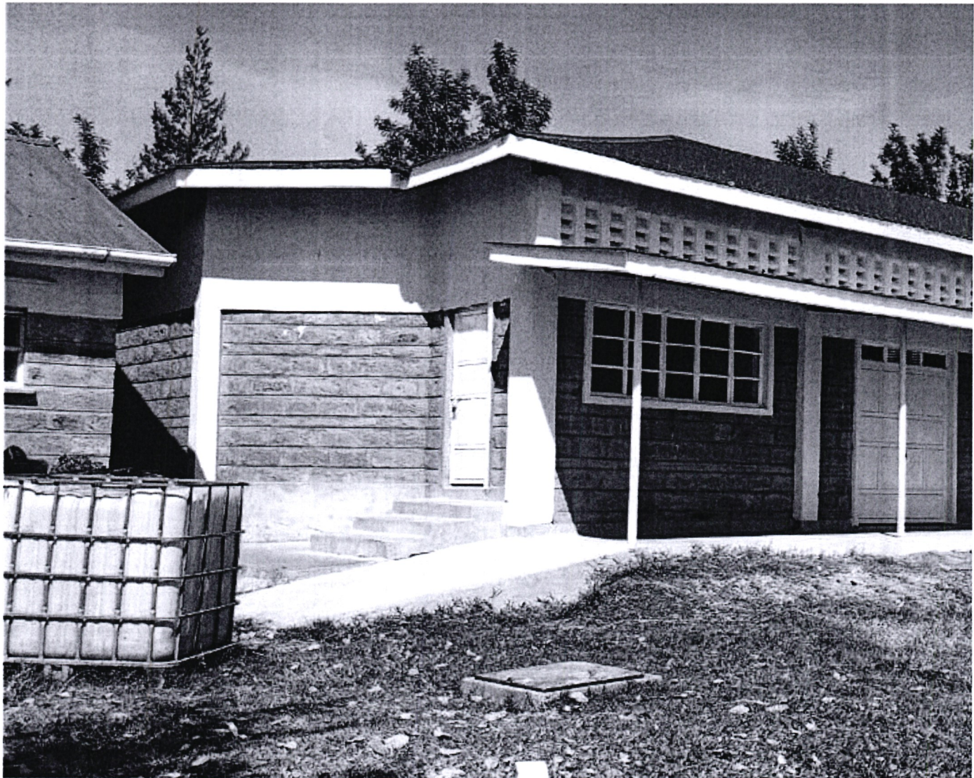
Fig 1: construction of a dining hall at Kibos secondary school.
