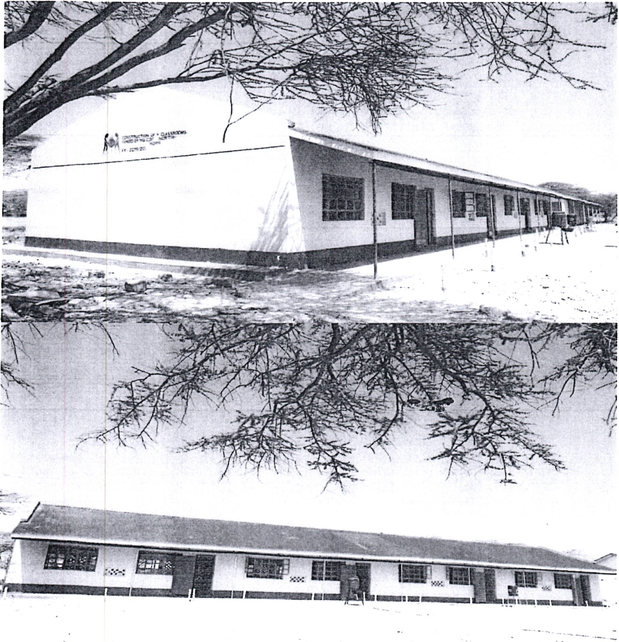
Figure 1 North Horr Boys Secondary School - Construction of 4 classrooms to completion
