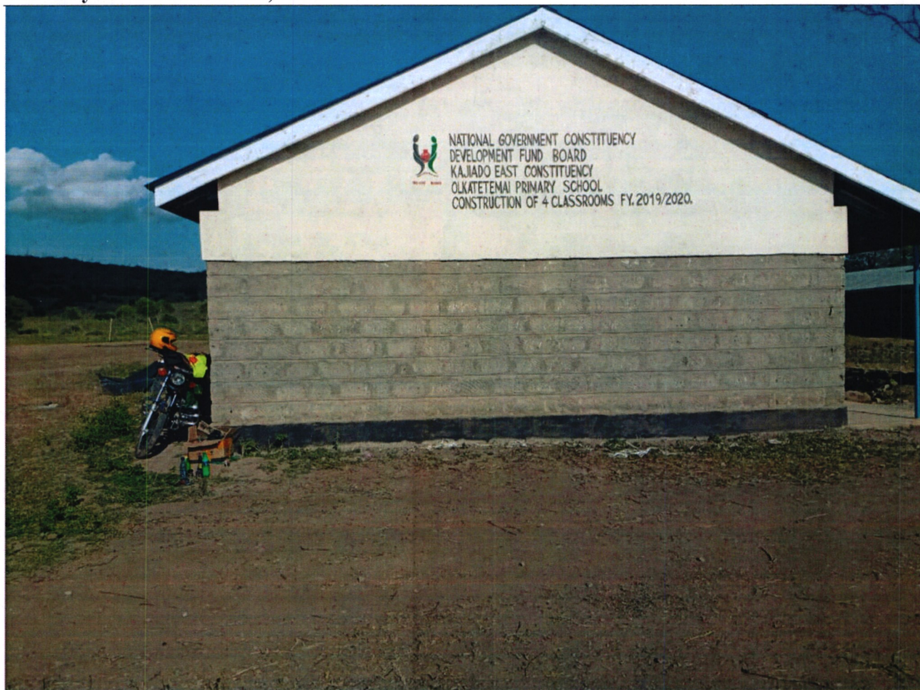
Olkatetemai primary school construction of 4 classrooms.
