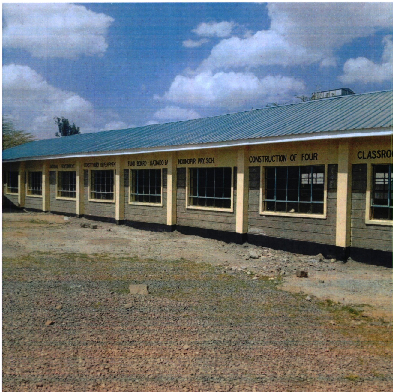
Noonkopir primary school construction of 4 classrooms.
