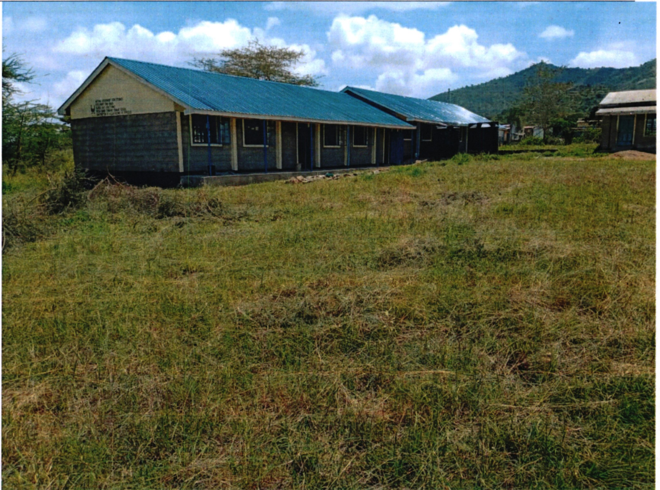
Sultan Hamud township primary school construction of 4 classrooms.
