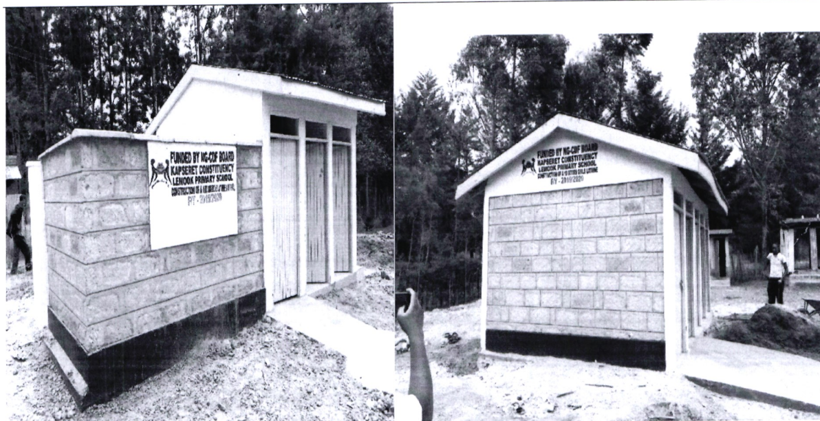
Complete 6no. Doors Boys pit latrine with urinal at Lemook Primary School and Complete 10no. Doors Girls pit latrine at Lemook Primary School.
