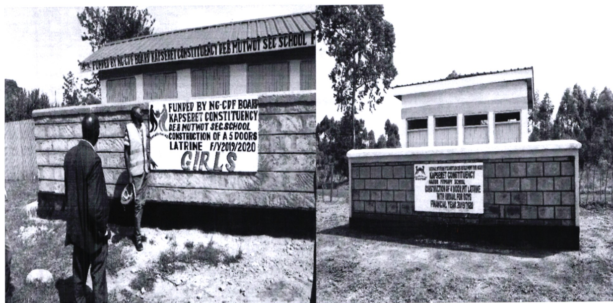
Complete 5no. Doors Girls pit latrine at DEB Mutwot Secondary School and 4 no. Doors Boys pit latrine with urinal at Nairiri Primary School completed respectively.
