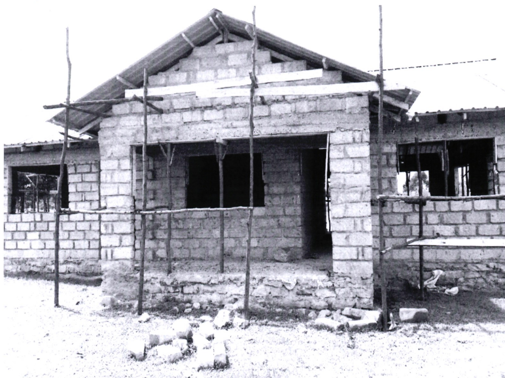
Ongoing construction of Administration block at Davies Secondary school.
