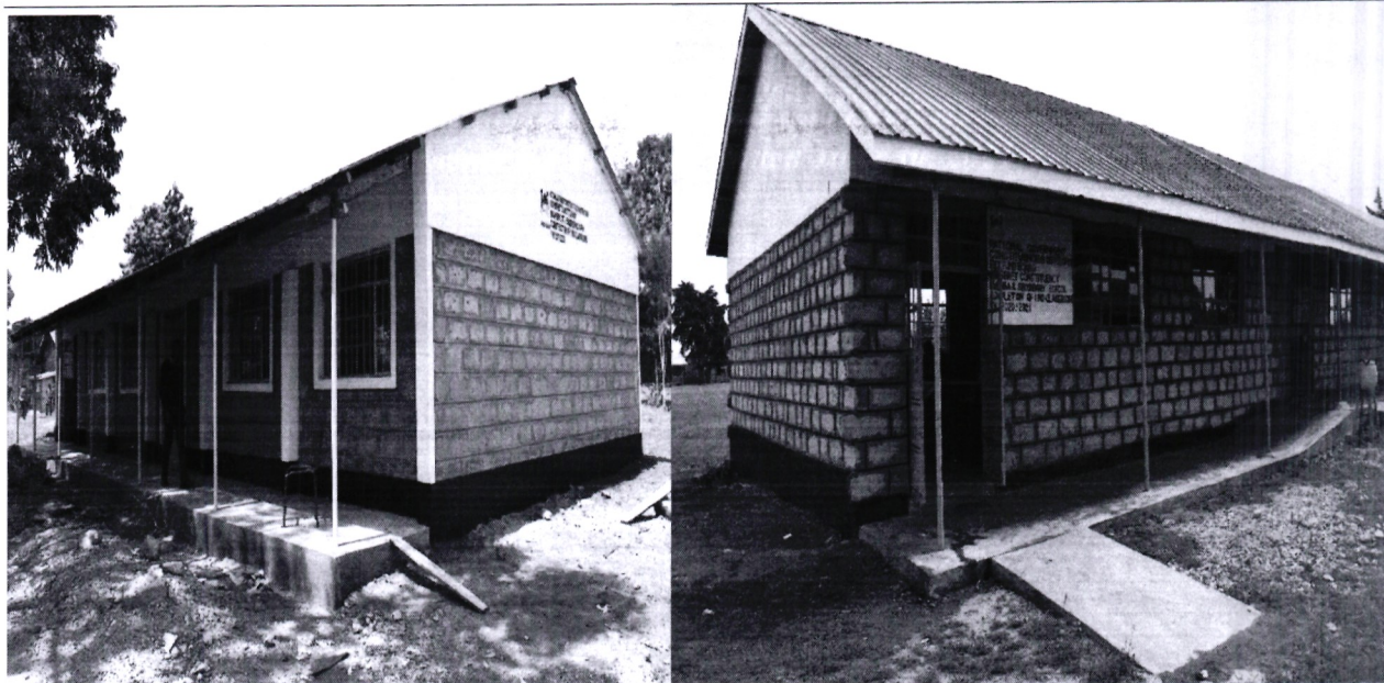
Complete 2no. Classrooms at Mwirutu Secondary School and Complete 1 no. Classroom at Kiambaa Secondary School respectively.
