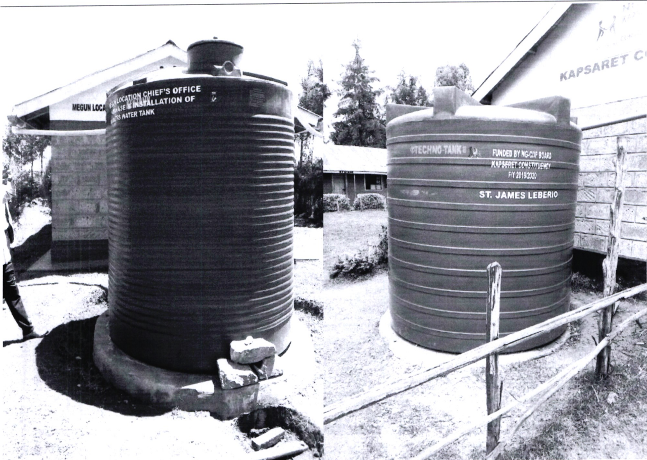
Complete Installation of 10,000 liters water tank at Megun chief's office and St. James Leberio Primary School.
