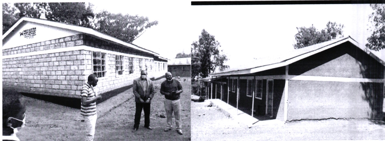
Before and after complete renovation of 8no. Classrooms at Tuiyobei Primary School.
