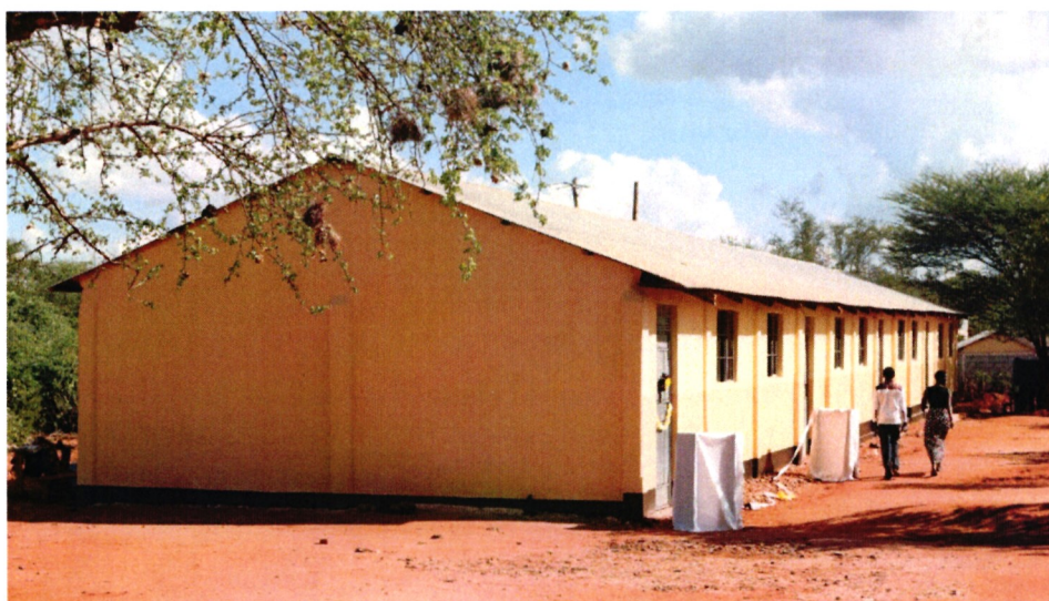
The new block that houses four classrooms constructed by the JKUAT Christian Union.
