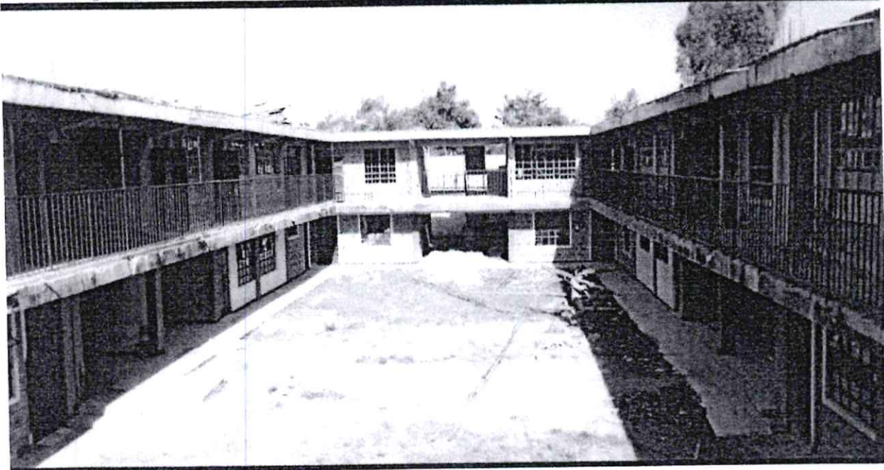
Ongoing Three 3No. Storey building at Sisenye Mixed Secondary school at Bunyala North Ward
