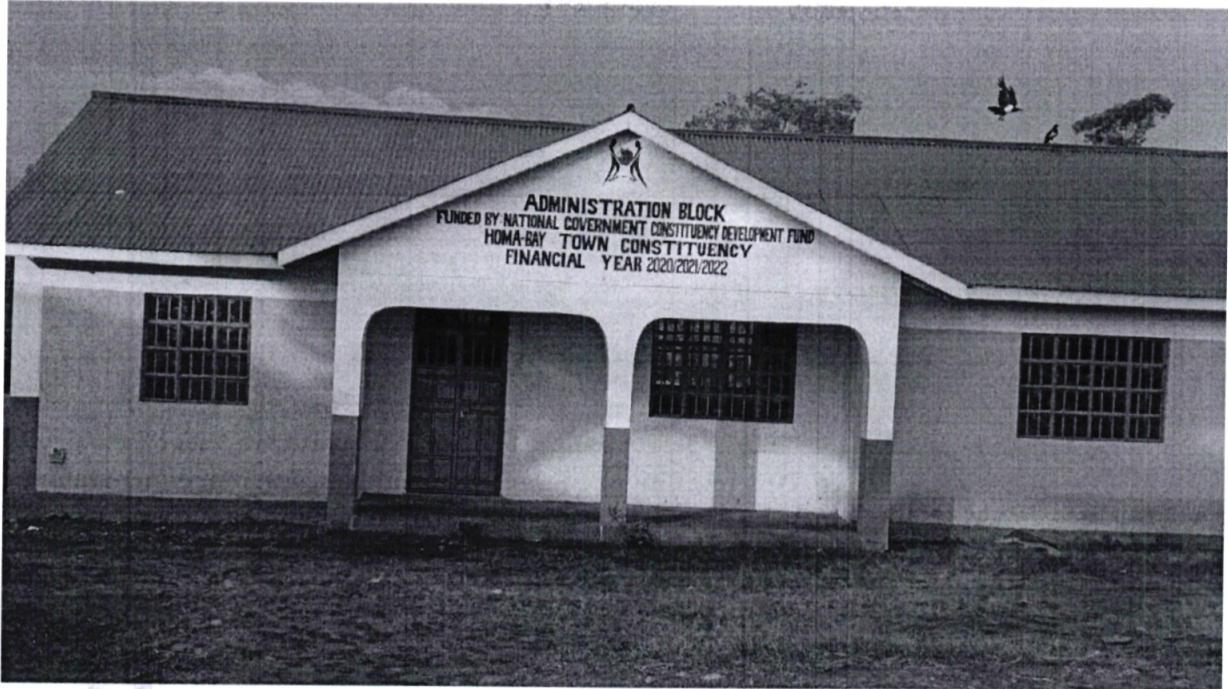
RODI PRIMARY SCHOOL: Completion of Administration Block
