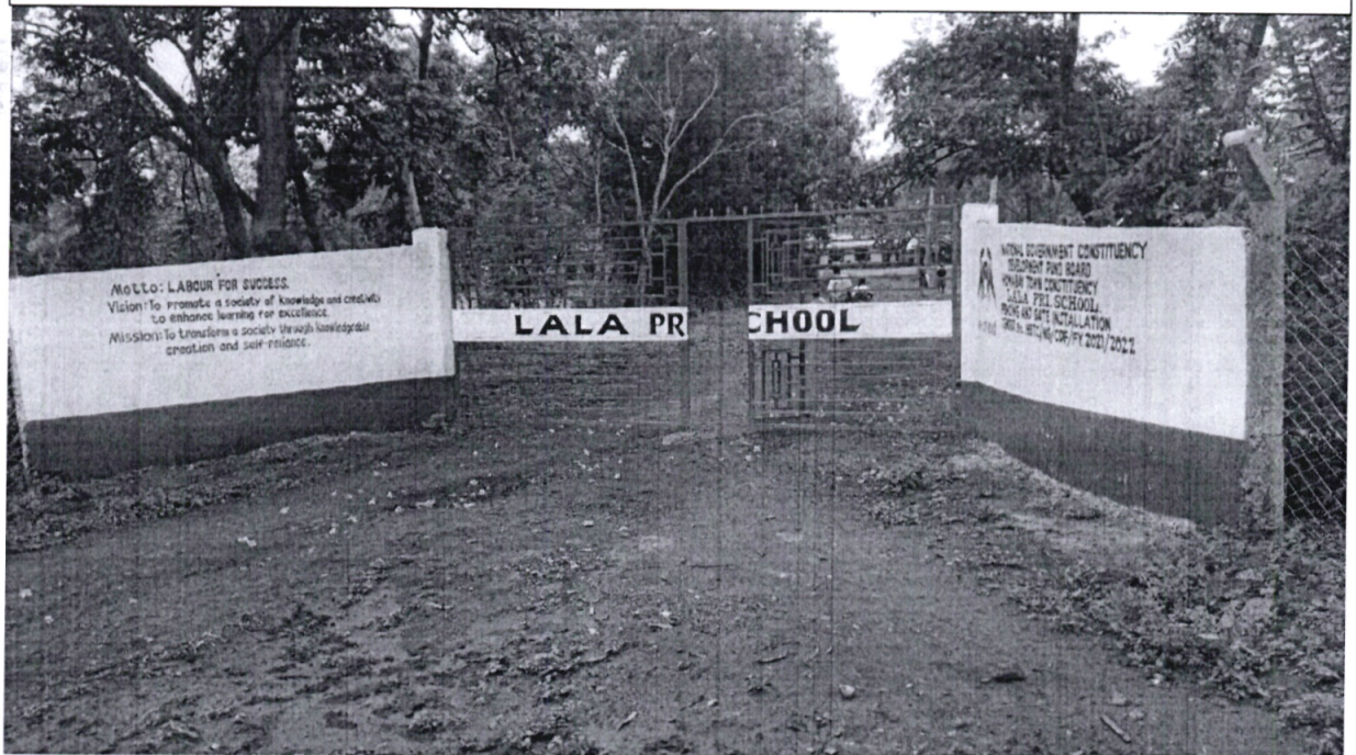
LALA PRIMARY SCHOOL: Gate installation and fencing of 6 ha. School compound
