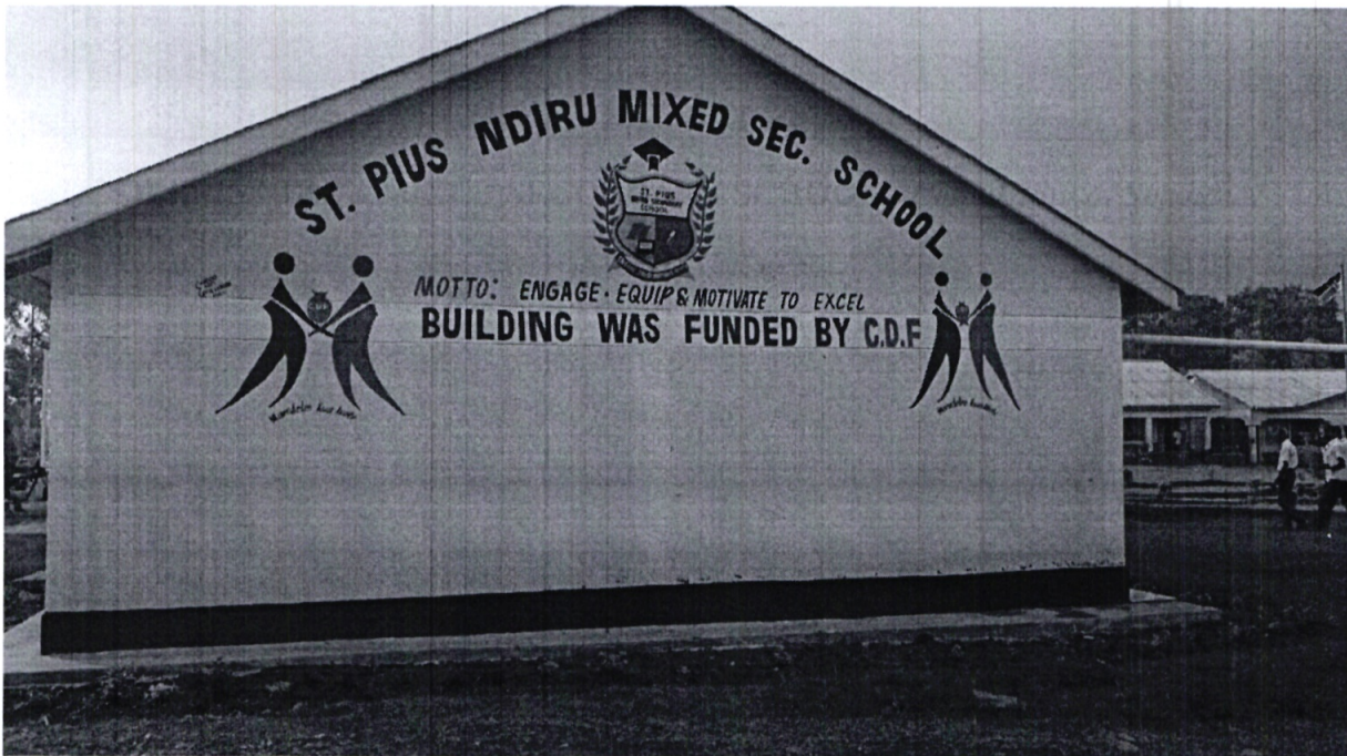
ST. PIUS NDIRU MIXED SECONDARY SCHOOL : Completion of Science Laboratory Side View
