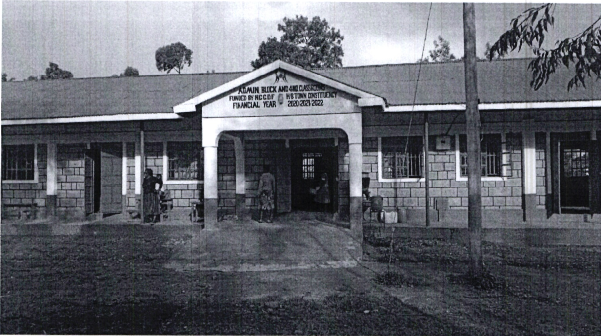
LORATENG PRIMARY SCHOOL: Completion of 4no. Classrooms and Administration Block
