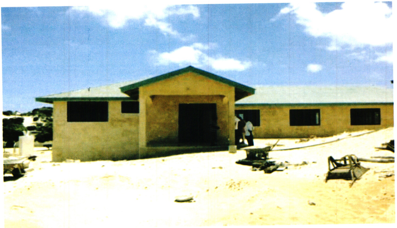
Construction of library at Bright Girls Secondary School
