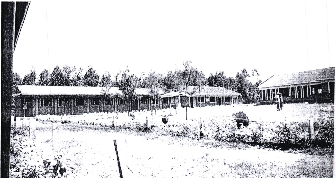
FIG 3 Shows a newly constructed laboratory and classrooms at Mikuva Secondary School in the financial year 2017 – 2018 Webuye East Constituency for enhancing learning environment.
