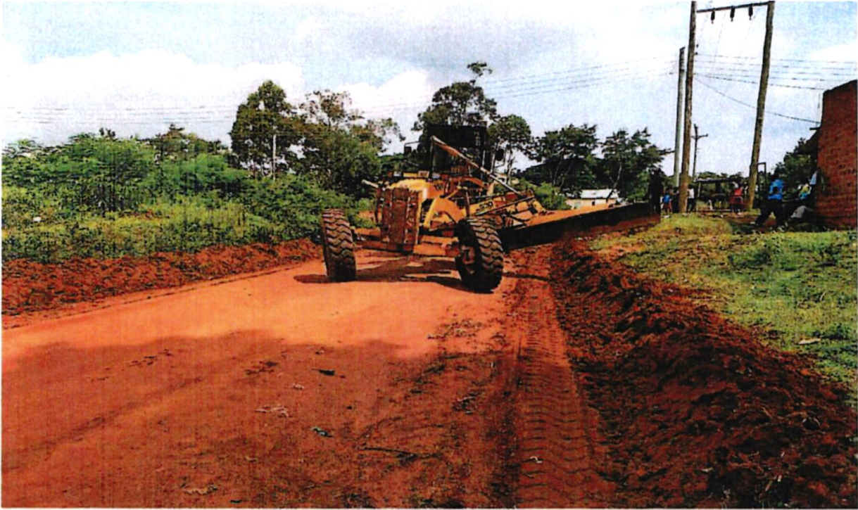
Routine Maintenance of Gravel Roads within the County
