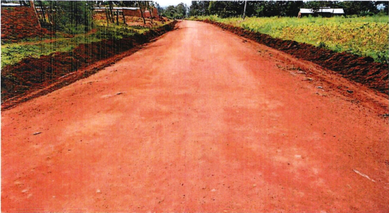
Routine Maintenance of Gravel Roads within the County
