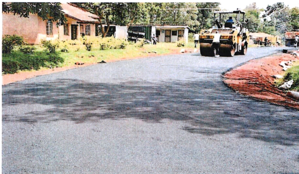
Upgrading of Road Infrastructure in Busia Municipality to Bitumen Standard
