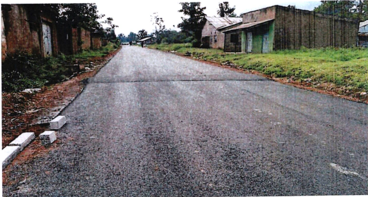
Upgrading of Road Infrastructure in Busia Municipality to Bitumen Standard
