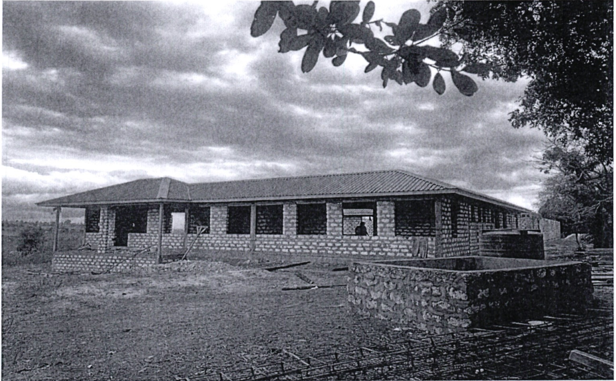
On-going construction of Mombasa GBVRC centre at Mwakirunge in Kisauni Constituency
