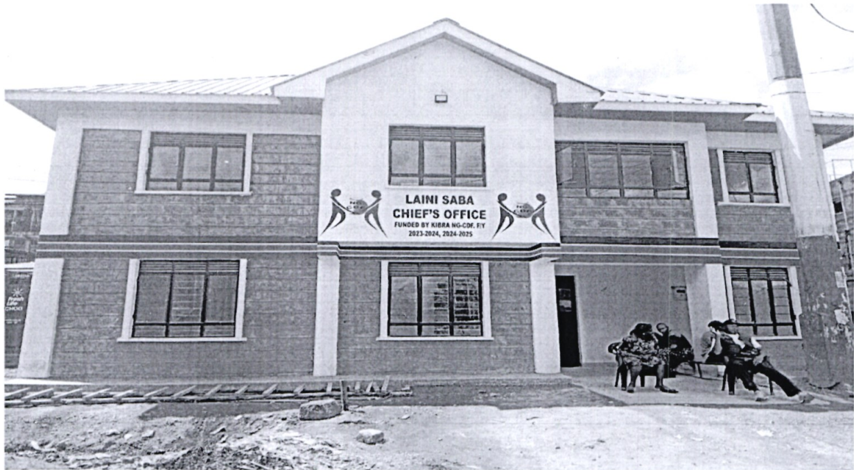
Fig 8: CONSTRUCTION OF LAINI SABA CHIEF'S OFFICE
