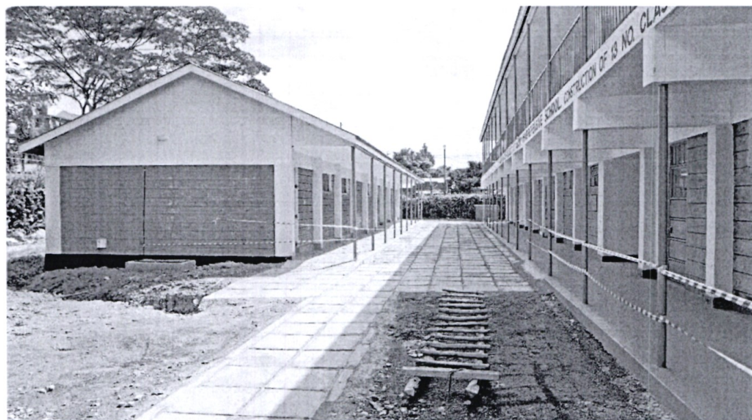
FIG 3: AYANY PRIMARY SCHOOL CONTRUSTION OF 13 NO. CLASSROOMS
