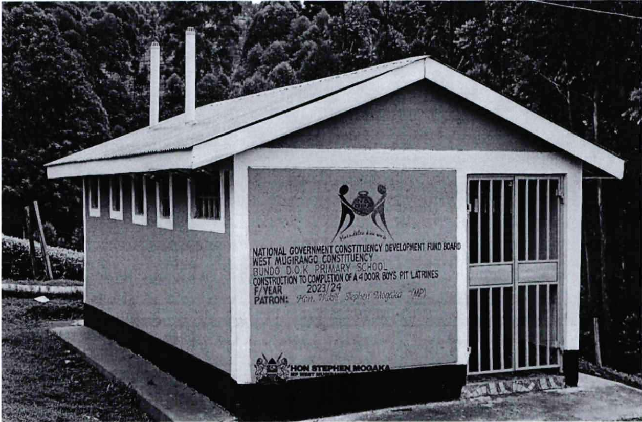
Pic 2: Bundo DOK Primary school; Construction of boy's pit latrine
