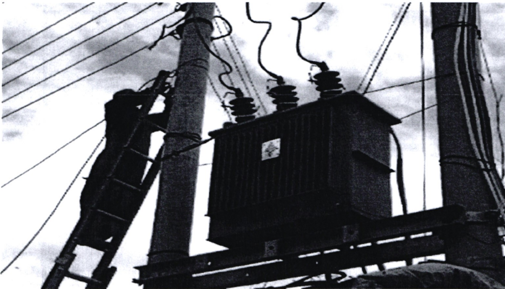
Figure 4.2.7-ii: Kenya power engineer at work- NMC produces transmission parts for Kenya power transformers
