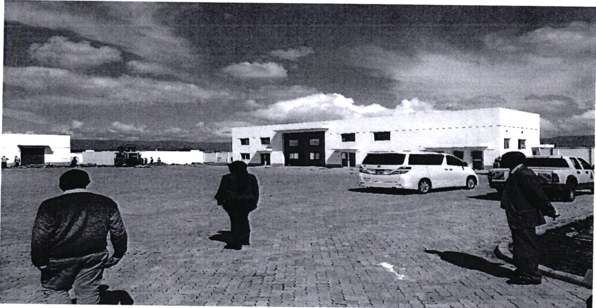
Figure 4.1.3-i: Internal Container Depot at Naivasha SEZ - Mai-Mahiu
