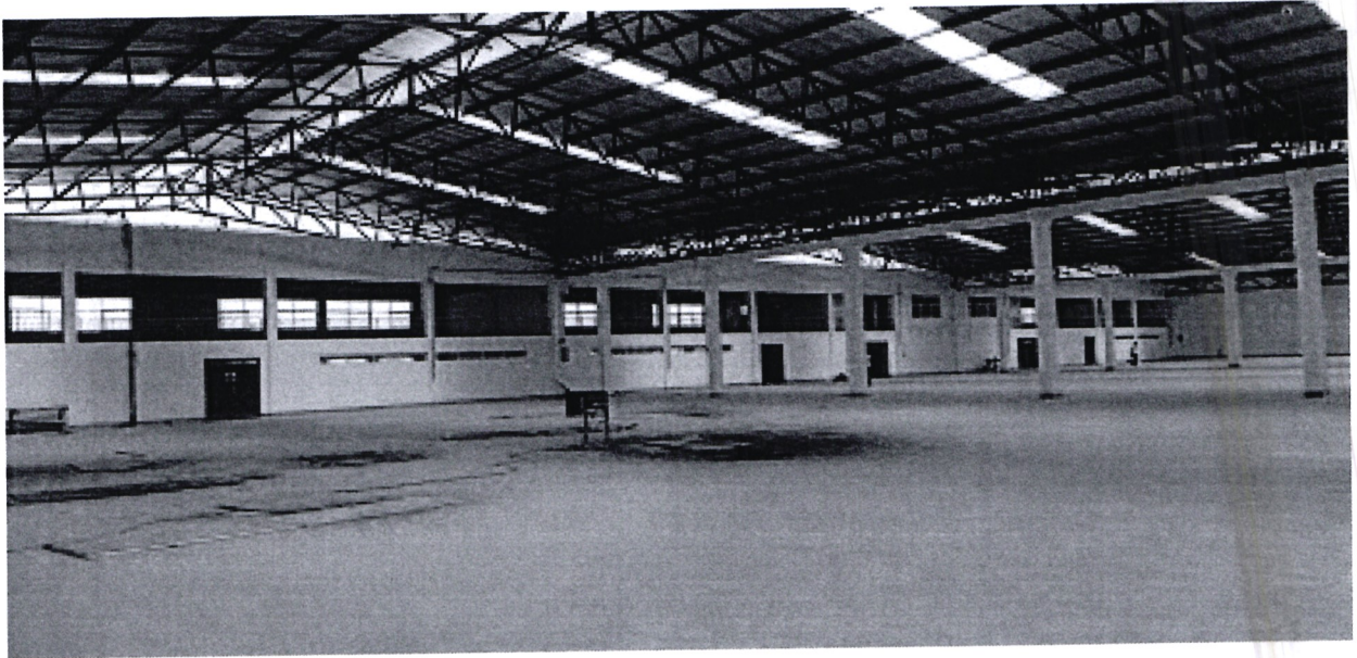
Figure 4.1.1-ii: Industrial Shed at EPZ, Athi River
