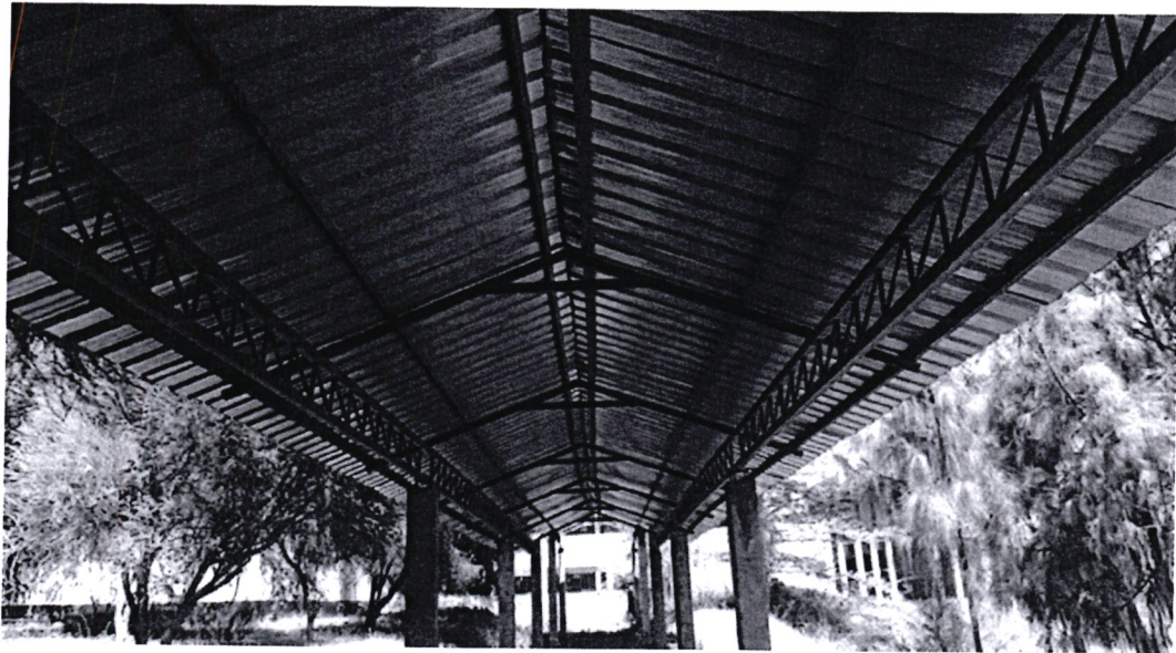
Figure 4.1.8-ii: Walkways at 90 % complete in KITI, Nakuru
