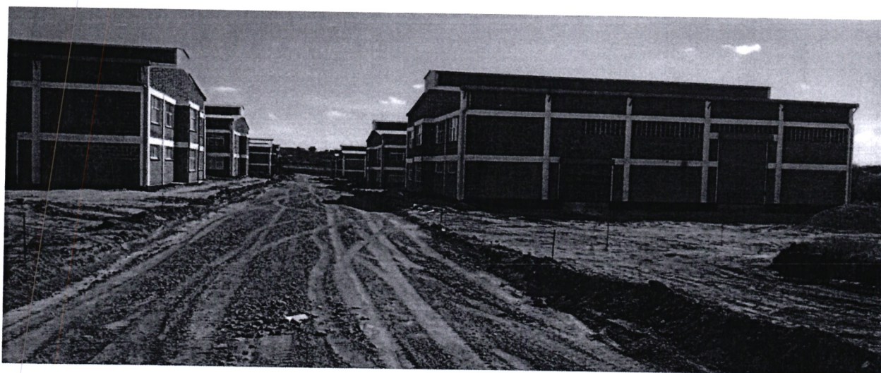
Figure 4.1.1-i: Road construction at EPZ, Athi River
