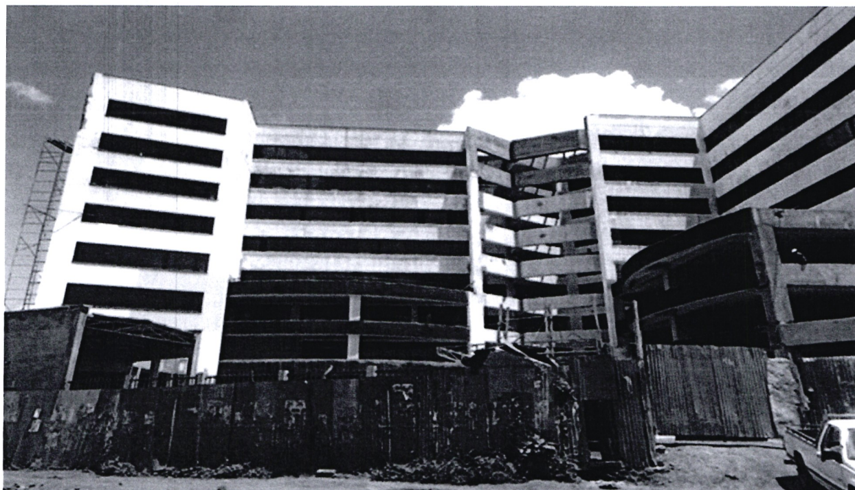
Fig. 27: KIBT Parklands office Complex currently under construction
