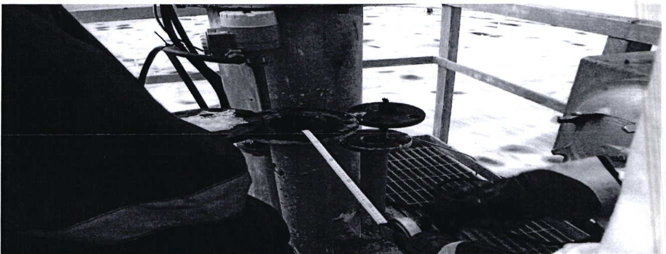
Fig. 19: Manual dipping point (gauge hatch) atop a storage tank – A demonstration of the old method of fuel Measurement that was replaced by the automatic tank gauging system
