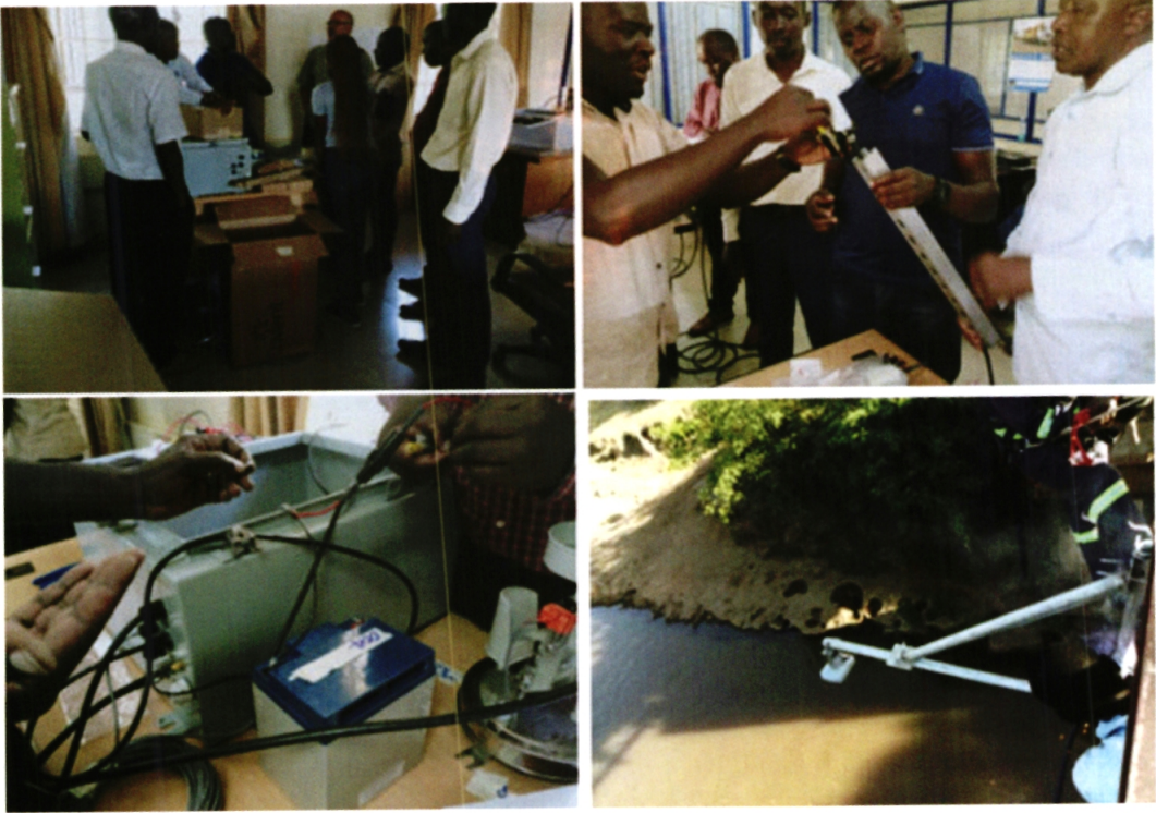
Figure 2.12: Bench testing and installation of hydromet equipment
