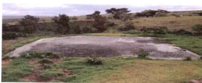
Raw sewer near prison houses - Nakuru
