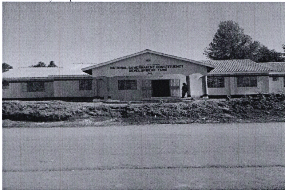
Construction of NGCDF office
