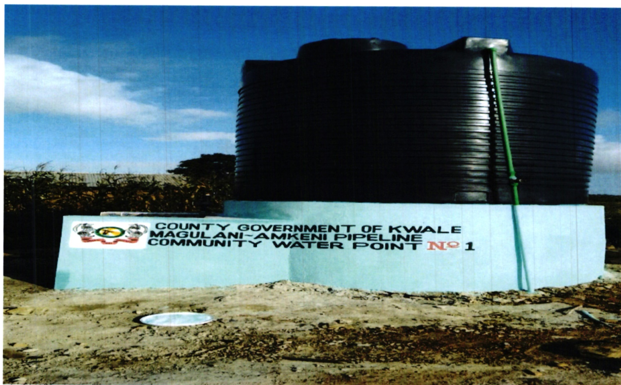
Magulani Amkeni Pipeline
