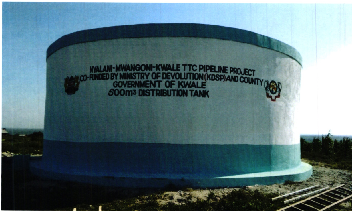
Nyalani Mwangoni Pipeline Distribution tank.
