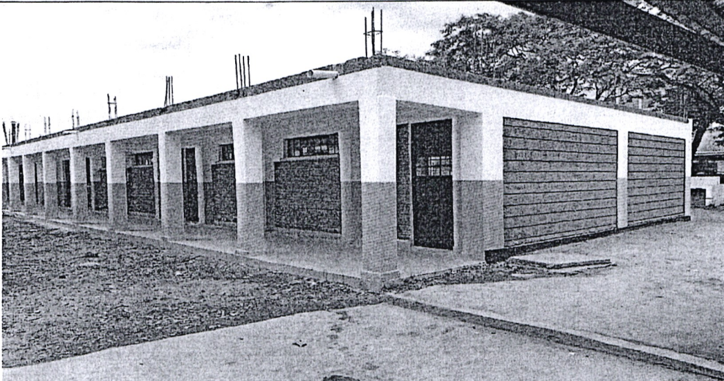
4 New classrooms at Aquinas High School
