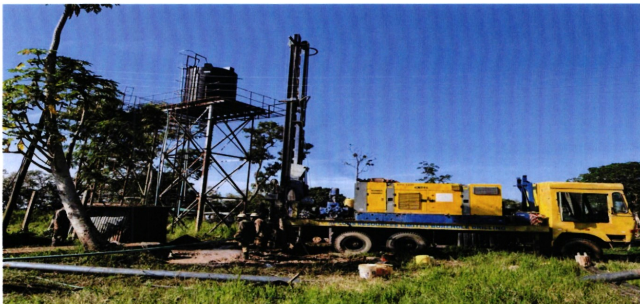
Drilling of a borehole
