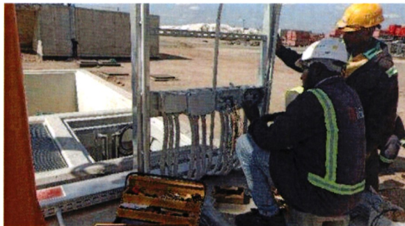
Filter feed pumping station -Pulling of armoured electrical and Trunking of cables
