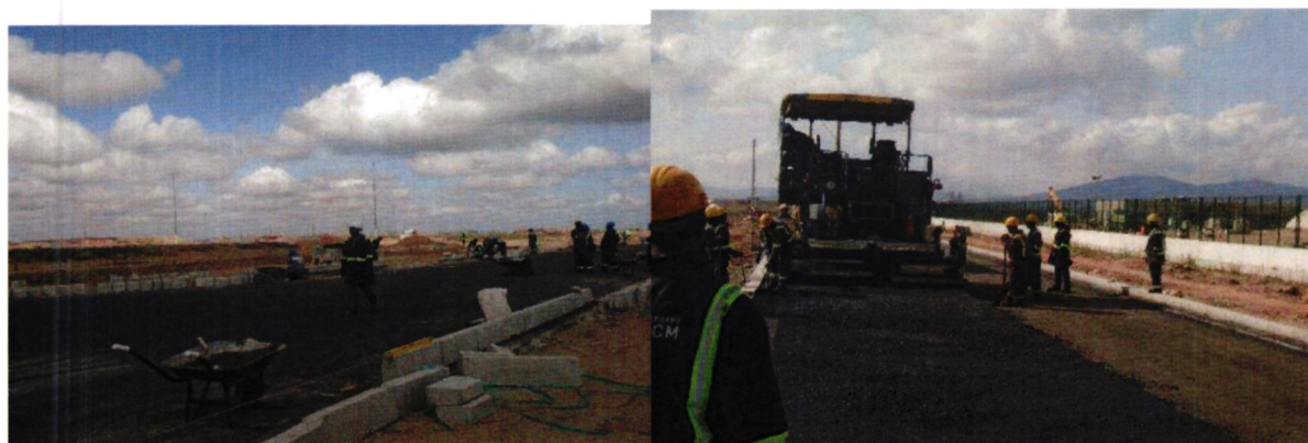
Hunching & installation of road kerbs on Auto Boulevard RHS and Laying of asphalt base course on WRF Road
