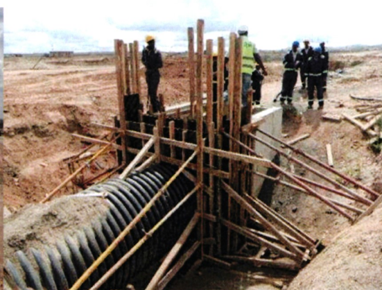
Formwork to manhole SD-05 Collar Along Auto Boulevard
