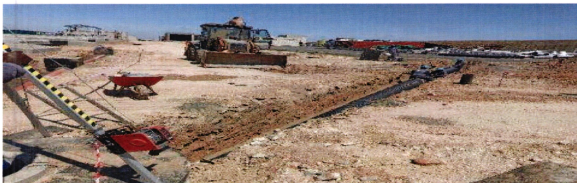
Conduit joining & alignment of stormwater process pipes along the Water Treatment Plant Road
