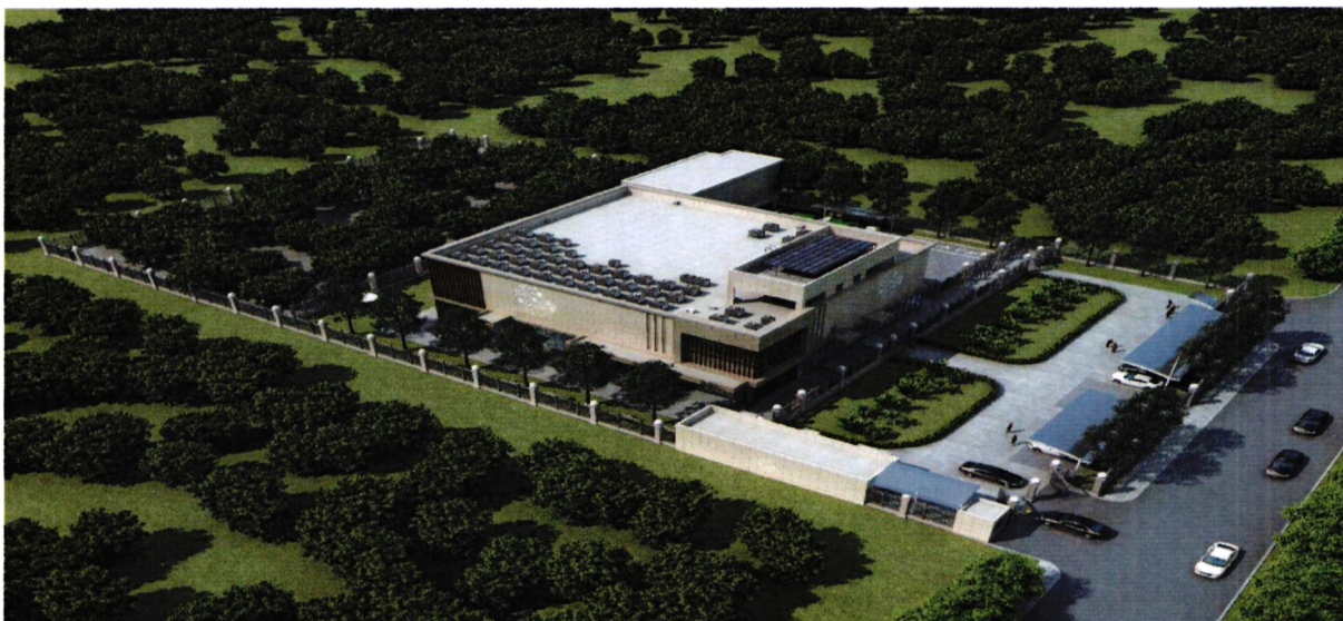
Illustration photo for the Data centre
