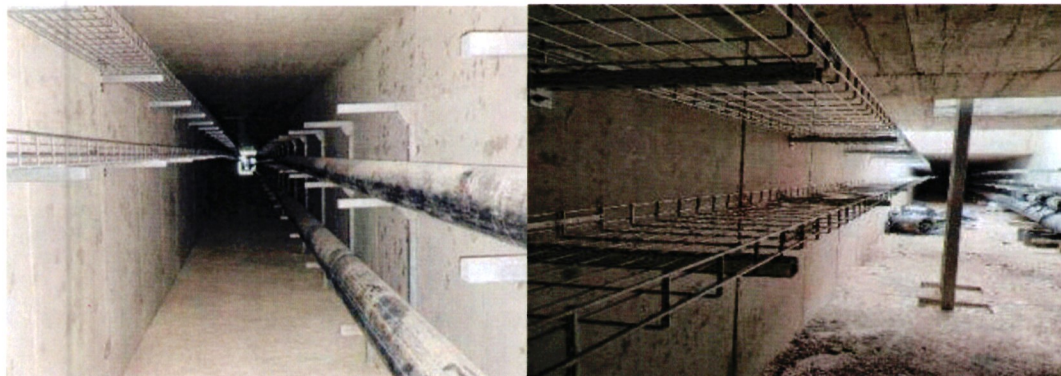
Section of Utility Tunnel in the Technopolis with HDPE pipes and support racks
