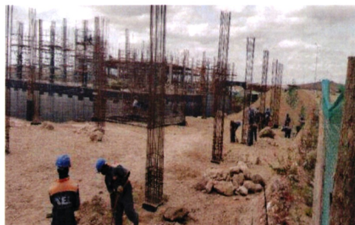
Living quarters - Backfilling work to formation level
