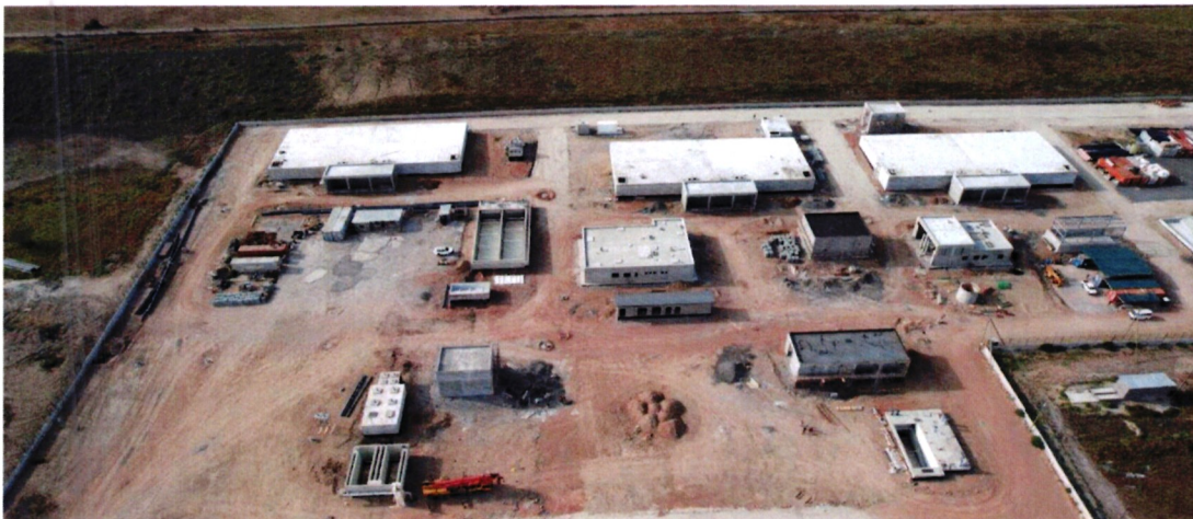
Arial view of Water Treatment plant
