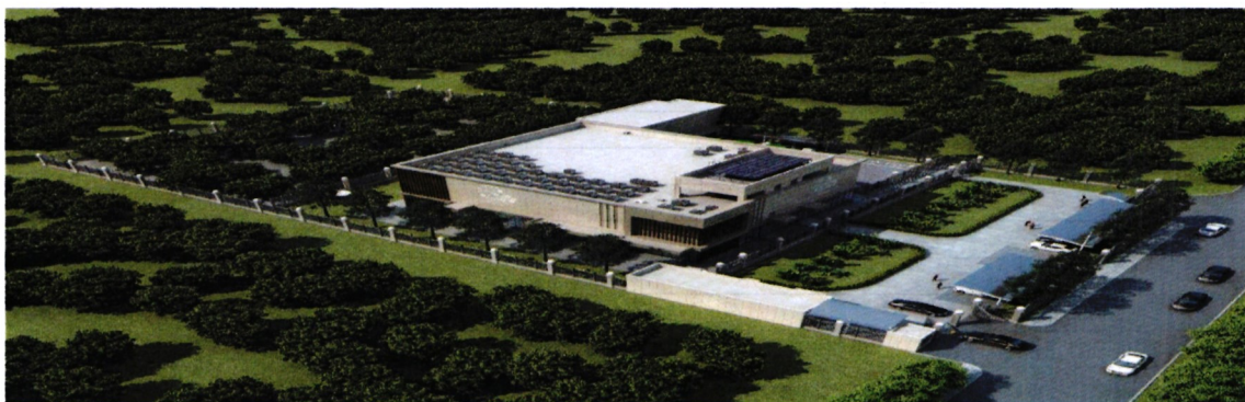
Illustration photo for the Data centre
