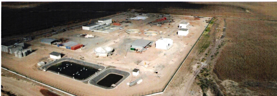
Ariel view of the wastewater reclamation facility
