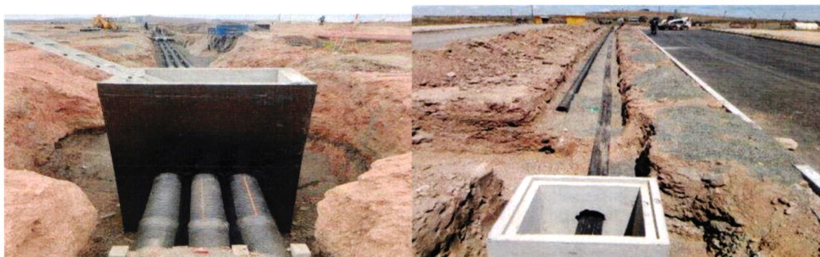
Sand bedding, conduit laying, backfilling, and installation of warning tape from LV-208 to LV-209 on Transit Road.
