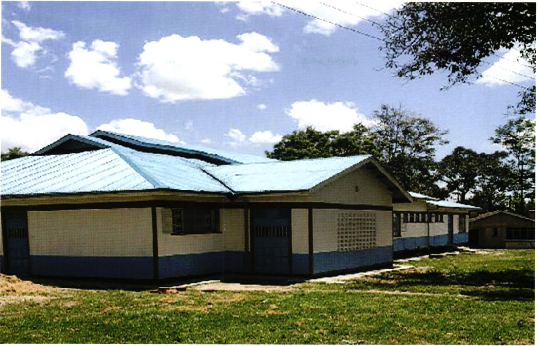
Theatre at Navakholo Sub-County Hospital, Kakamega County
