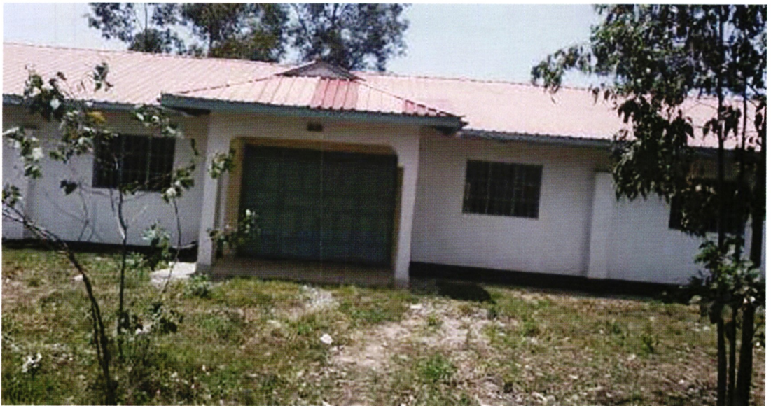
Construction of hostel at Sero Youth Polytechnic-Homa Bay County
