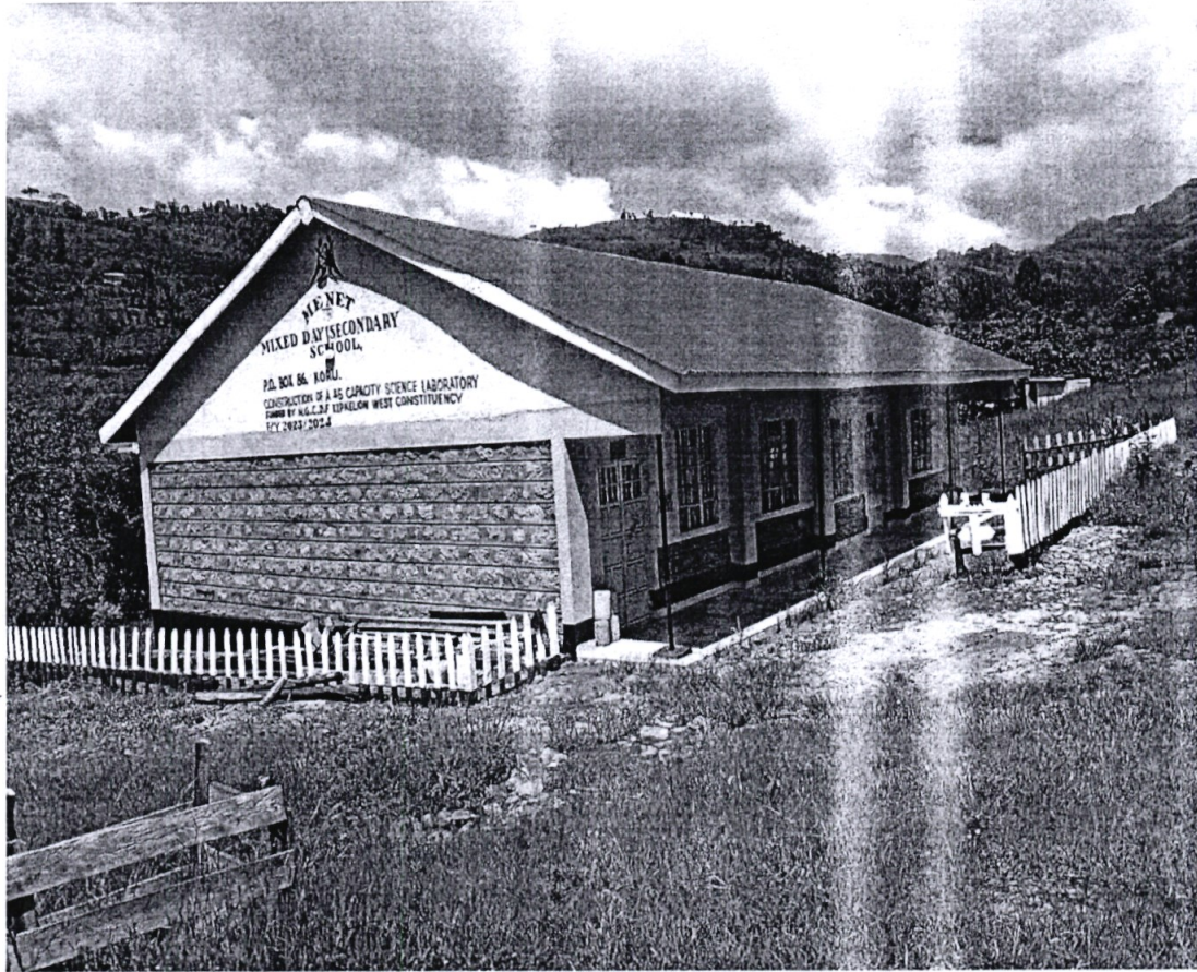
Menet secondary school construction to completion of single laboratory 45 capacity
