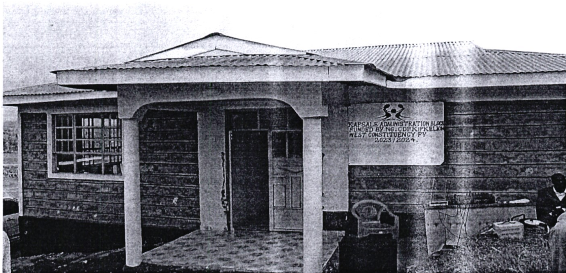
Completion of administration block at kapsale primary school
