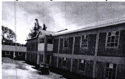
Construction of Dormitory at Kimasian Secondary school
