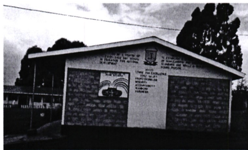
Construction of Laboratory at Londiani Township Sec. school
