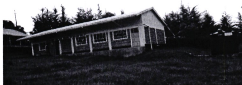
Construction of Classroom at Ringa Primary school
