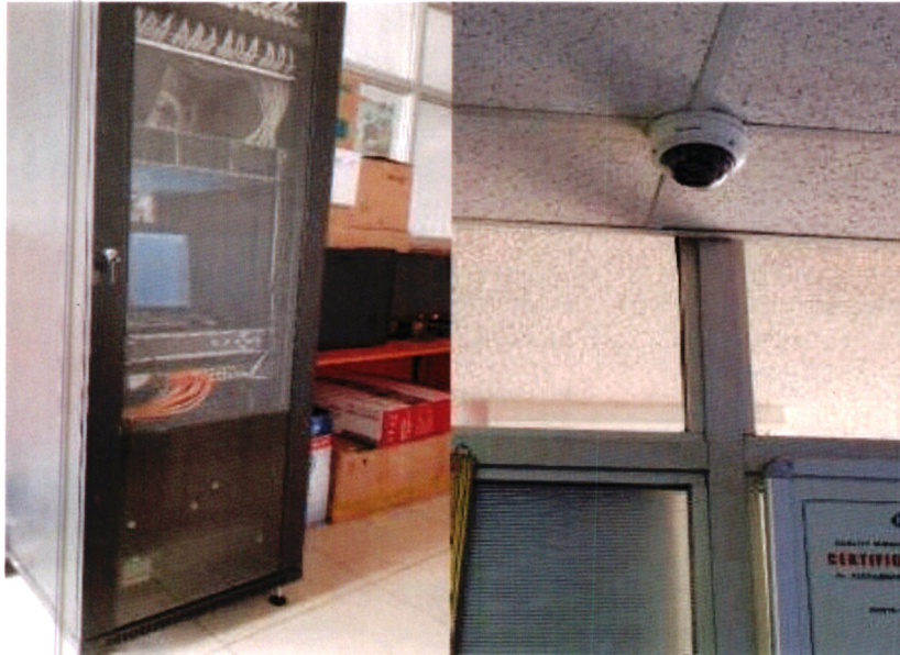
Installation of 42U server cabinet and CCTV cameras
