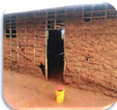
Infrastructural challenges, Grade 4 class-Maojo Primary School, Kilifi
