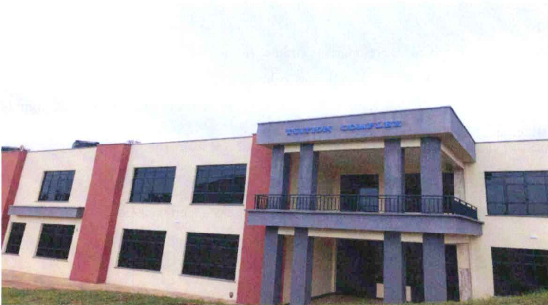
Tuition Block Phase 1 - ongoing
