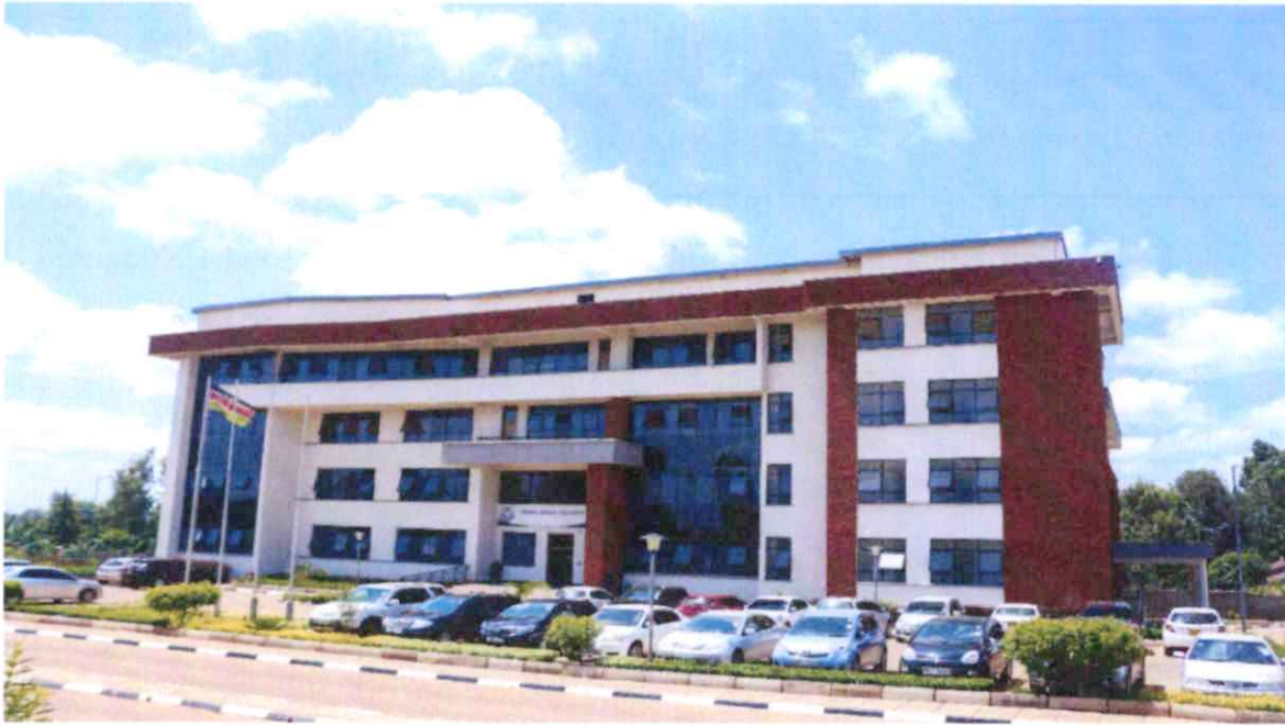
Administration Block – Awaiting final Accounts & Retention Refund
