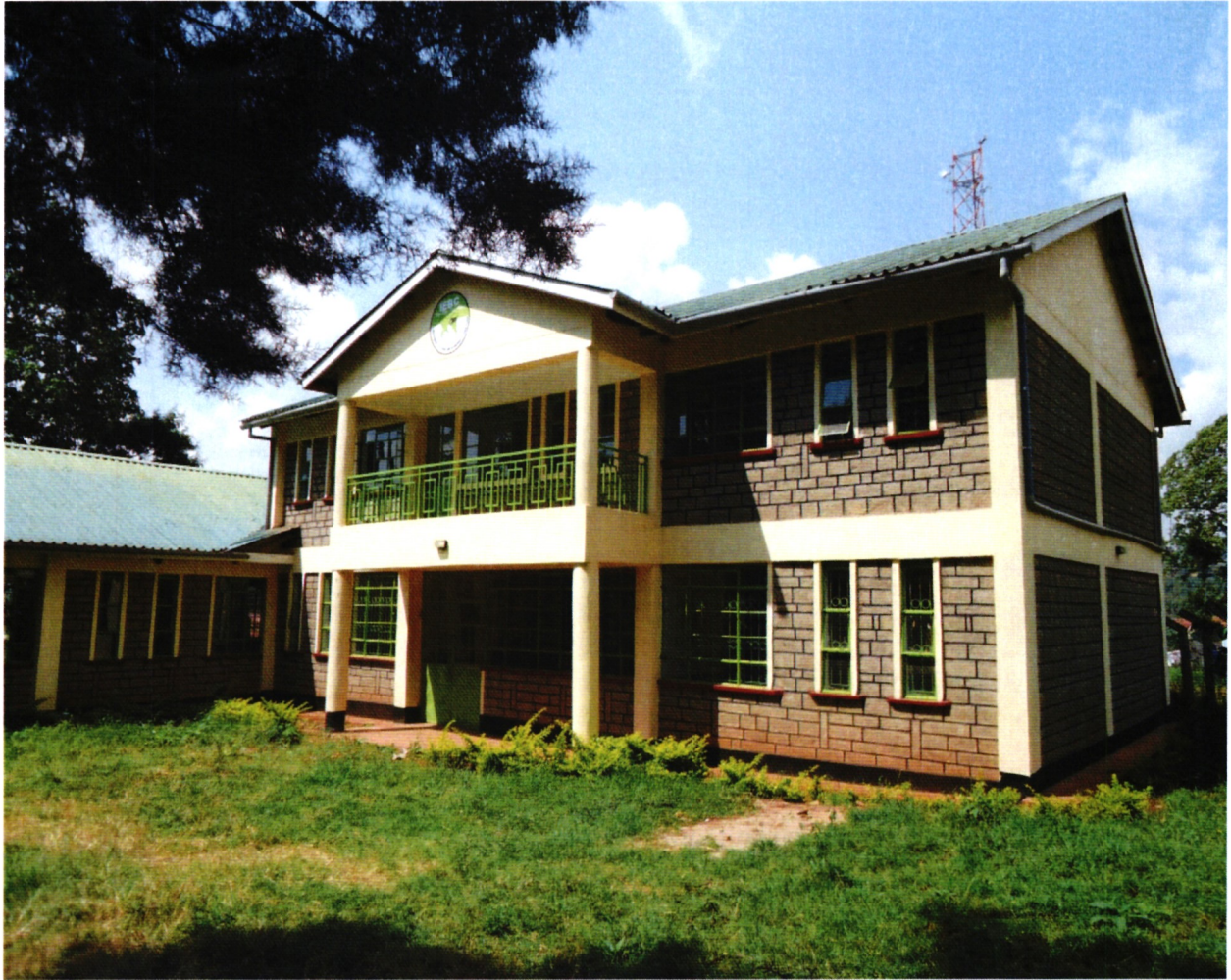
Newly Constructed Nyanza South Regional Office and Multipurpose Hall in Kisii County
