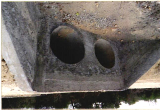
Marafa Chamari Road (culvert installation)
