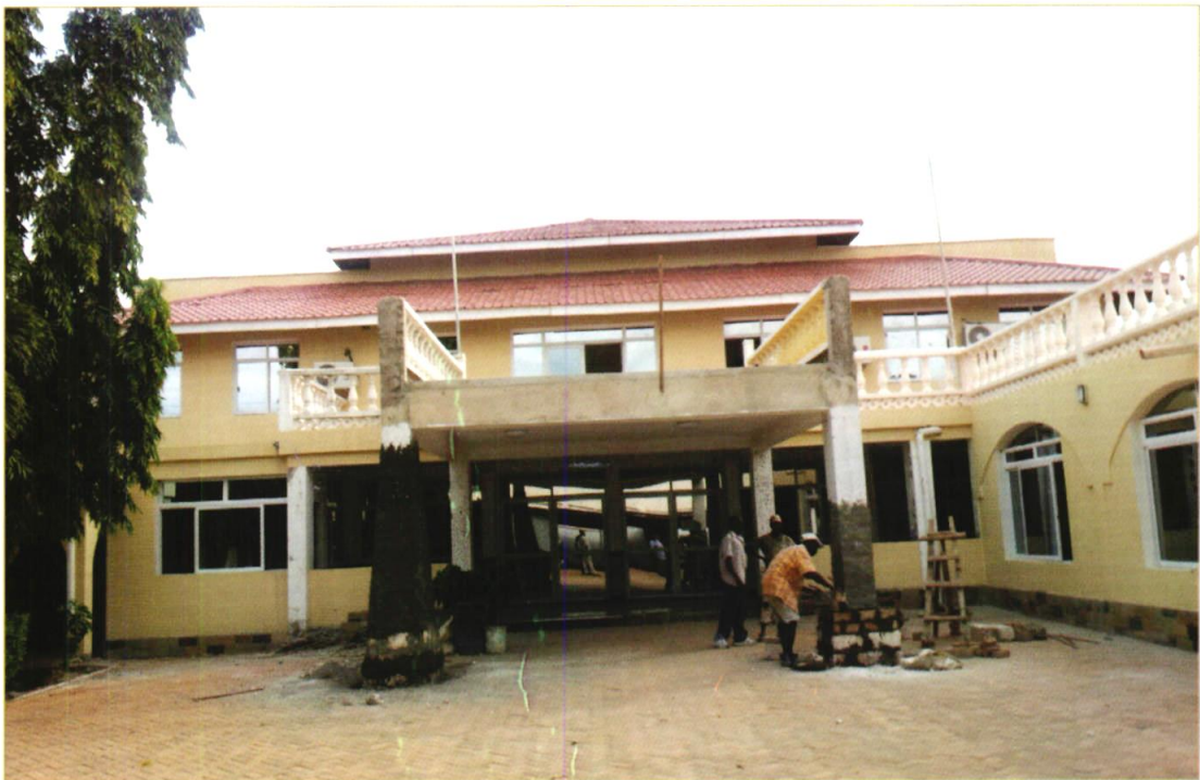
Kilifi Assembly Chambers under construction.
