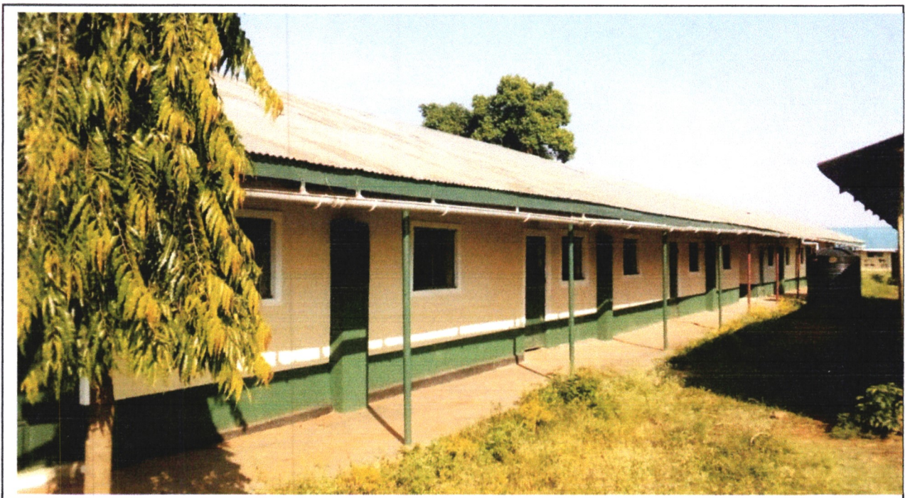
Wambarra Primary School 6 Classrooms
