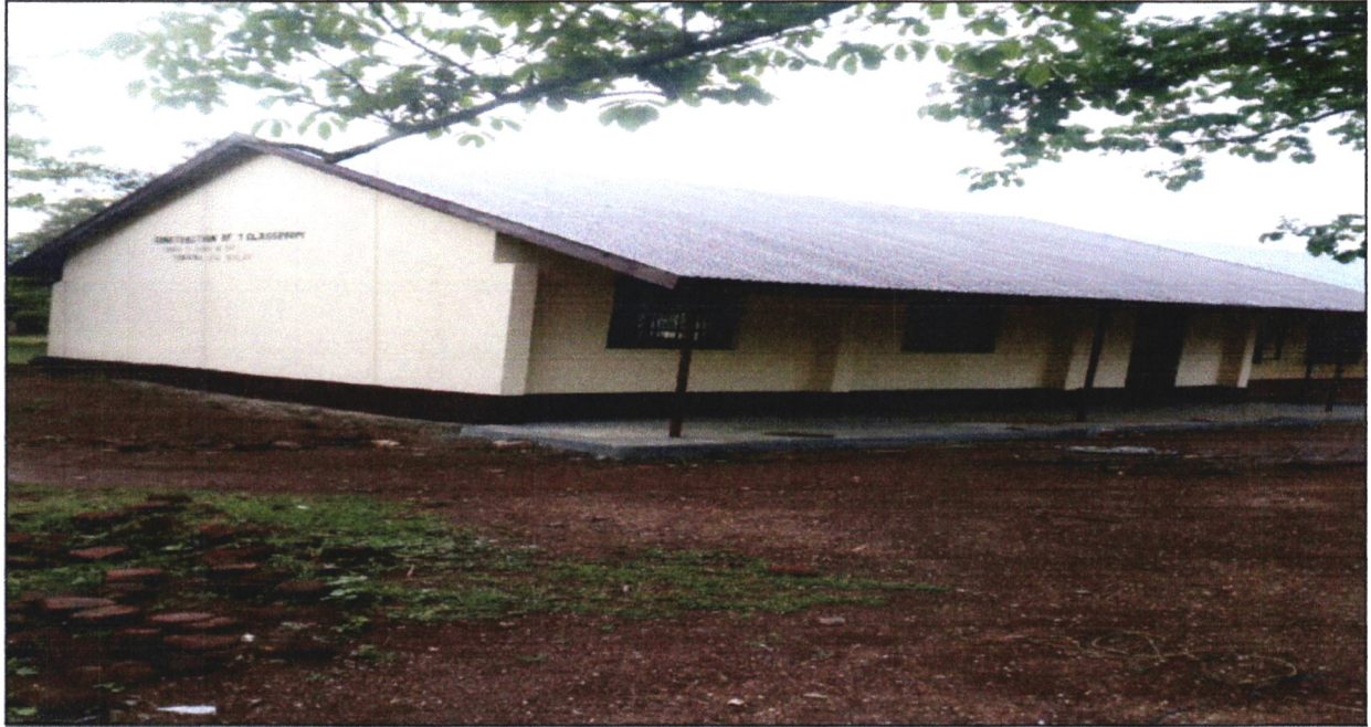
Mahanga Primary School Classrooms
