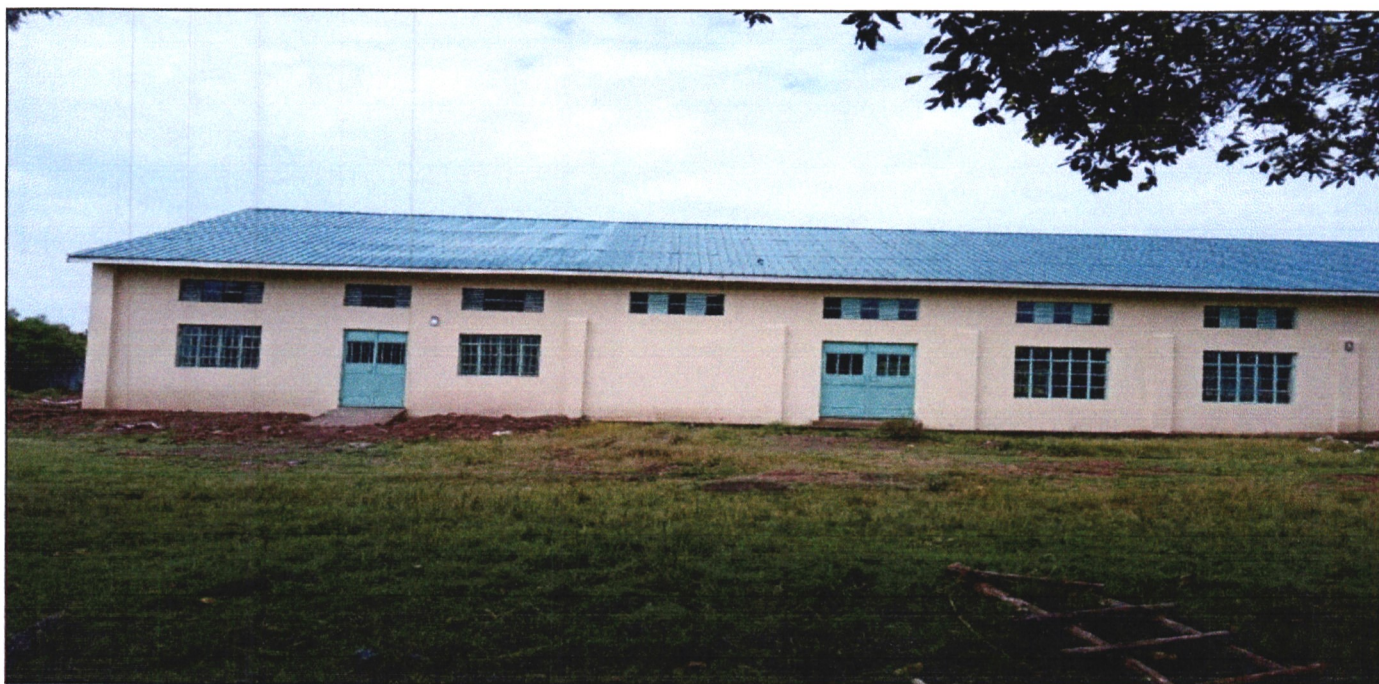
Majengo Secondary School Multipurpose Hall
