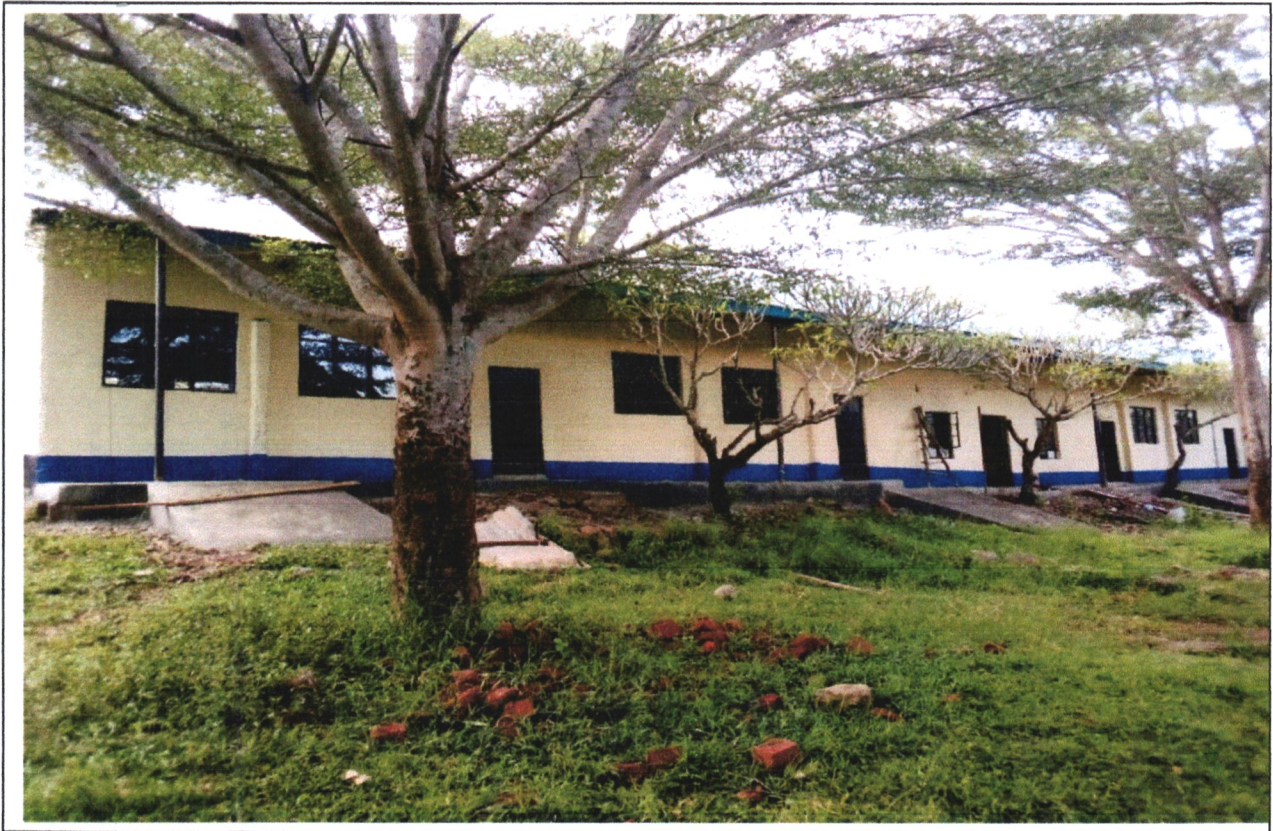
Kamnara Pry School 8 classrooms
