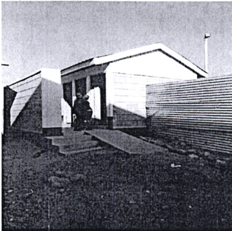
Figure 001: The project is complete but not labelled.
