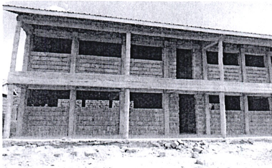
Figure 001: The front elevation of the classes The fixtures have not been installed.
