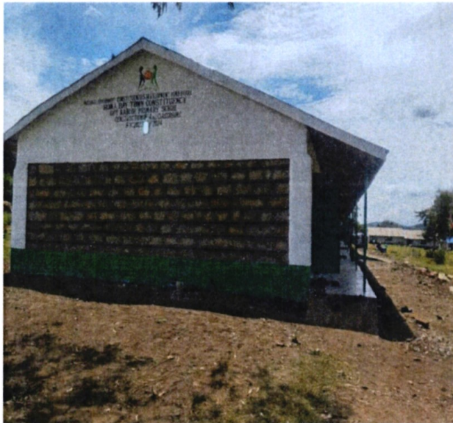
Got Rabuor Primary School- Construction of 4 classrooms at Kshs 5,000,000
