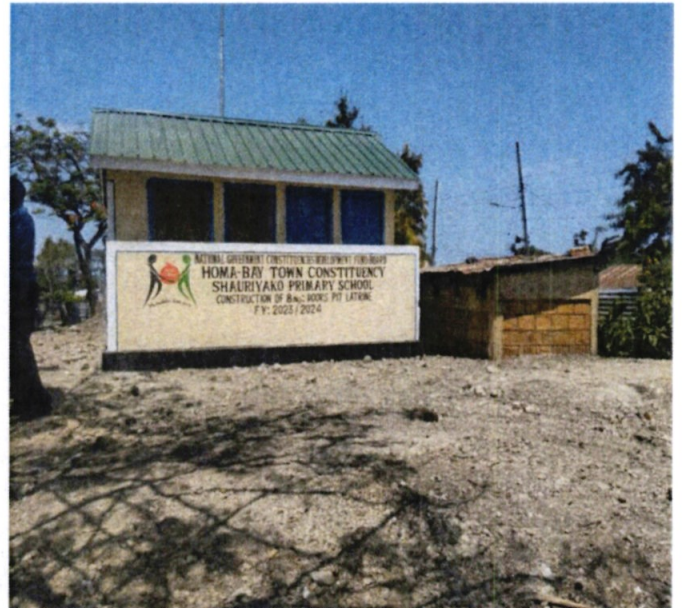
Shauri Yako Primary School - Construction of 8 doors pit Latrine at Kshs 1,200,000
