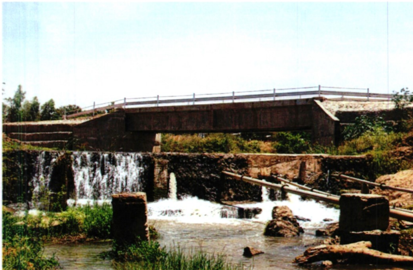
Ilviani primary access bridge
