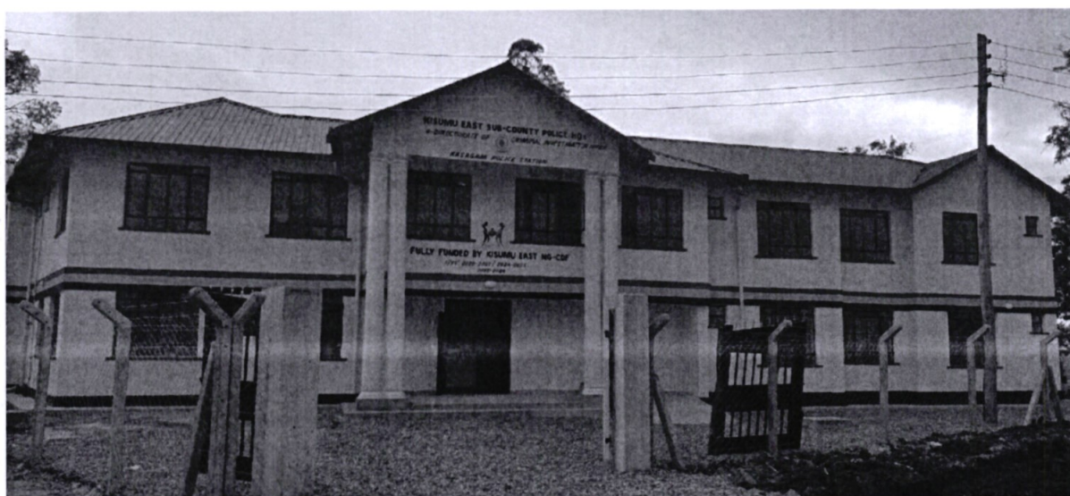
Figure 1: Construction of Kasagam Police Station
