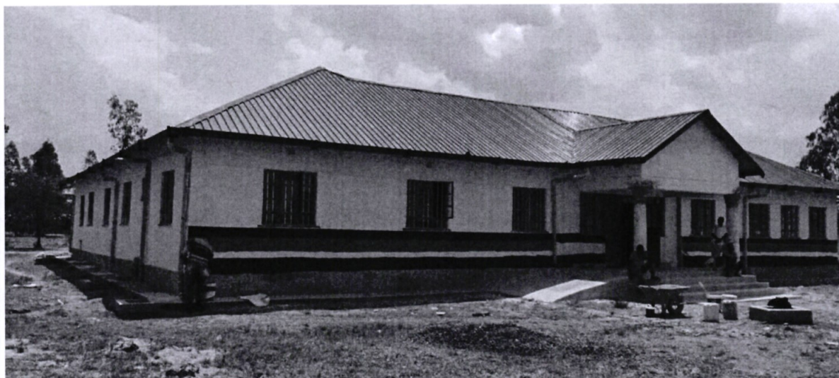
Figure 2: Construction of Chiga Police Station
