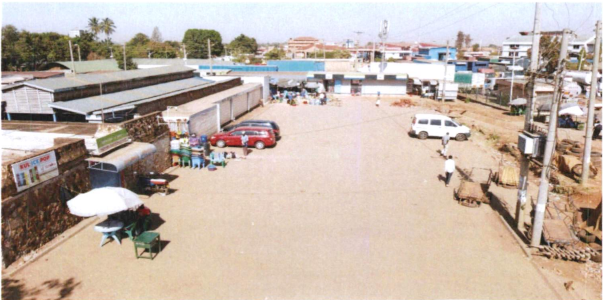
Newly laid cabros parking at the Taxi Park
