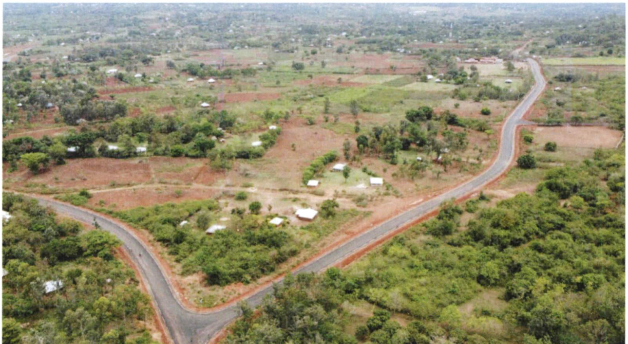
Newly tarmacked Bukiri-Mumbaka road
