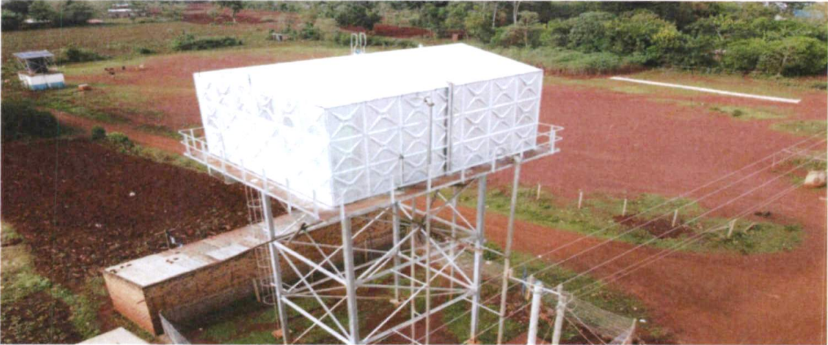
Rehabilitated Bumala overhead water tank
