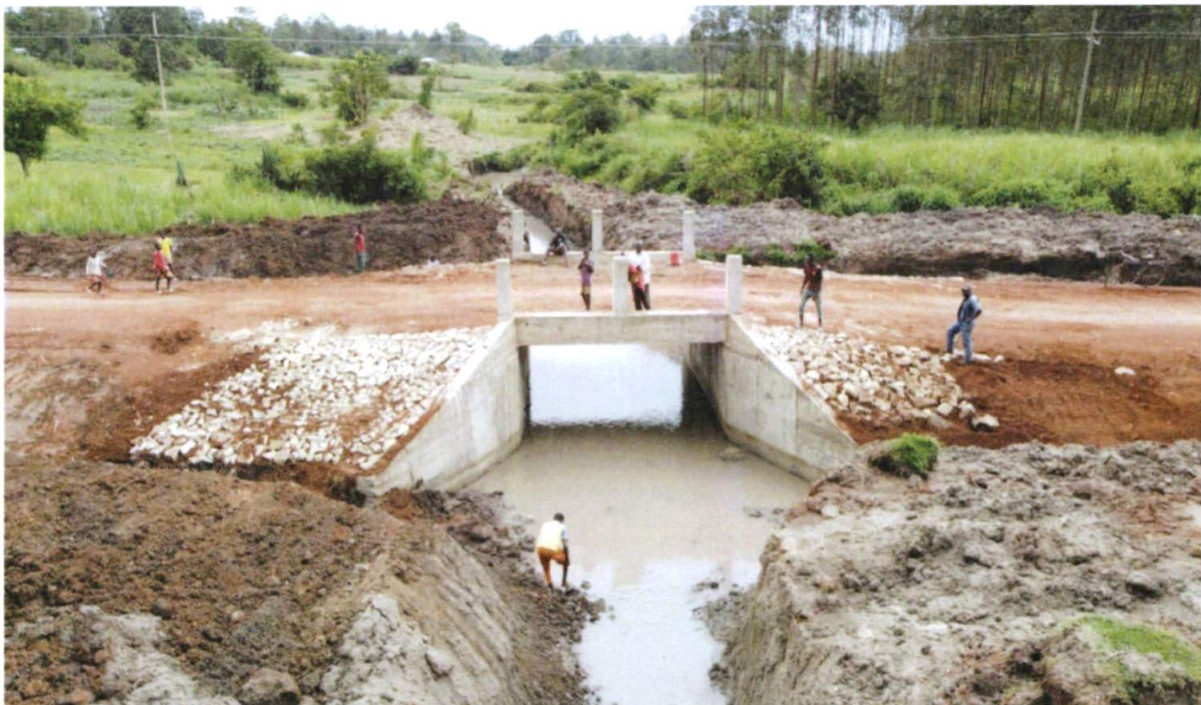
New Khayo bridge under construction in Nambale sub-county
