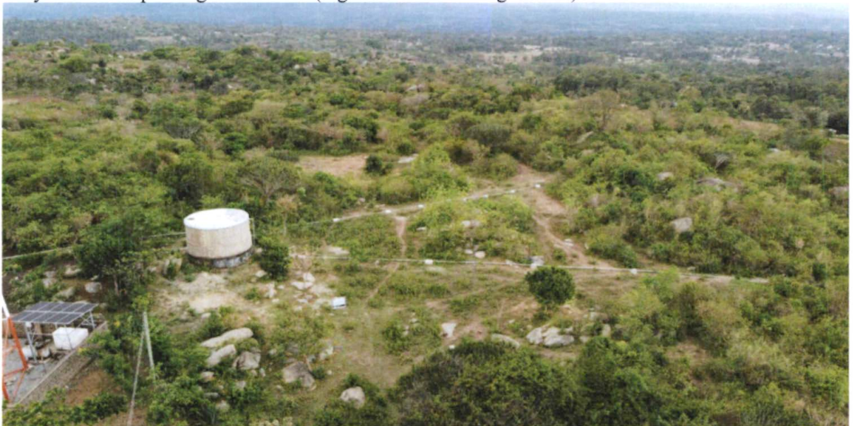
Installed water tank at Oshoromo hills
