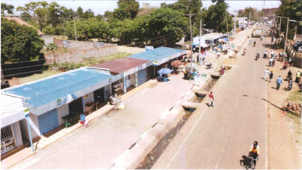
Newly laid cabros parking at the BCRH (Busia County and Referral Hospital)
