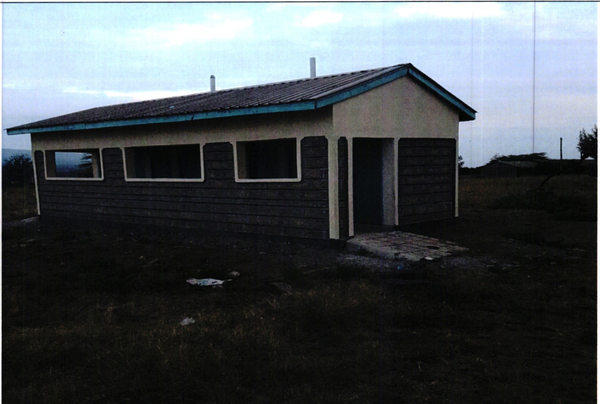
Olesharo Girls Secondary School Toilets- Ongoing painting works.
