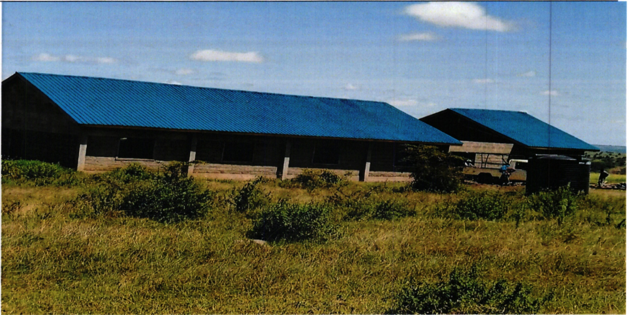
Olepunyua Primary School Ongoing construction of Dormitory
