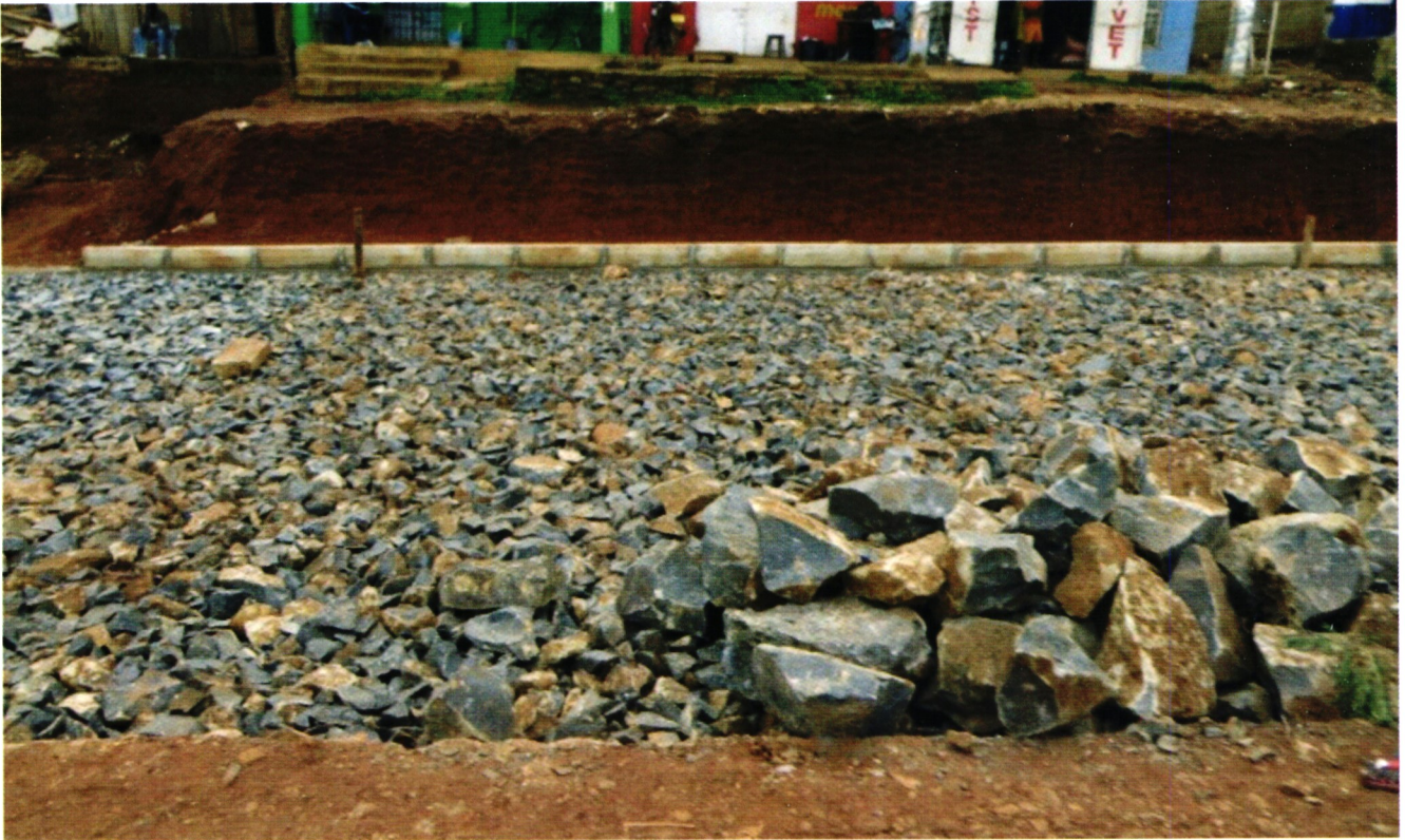
On-going road construction in West Pokot County.
