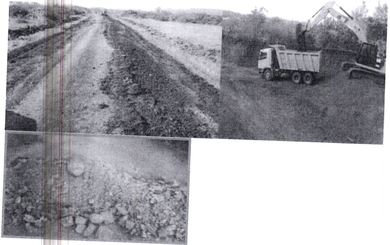
FIG 1.3 Grading and muraming of Okok-Kobodo-Kidoi-Malela road By NGCDF NDHIWA Constituency for Better transportation. FY 2017/2018
