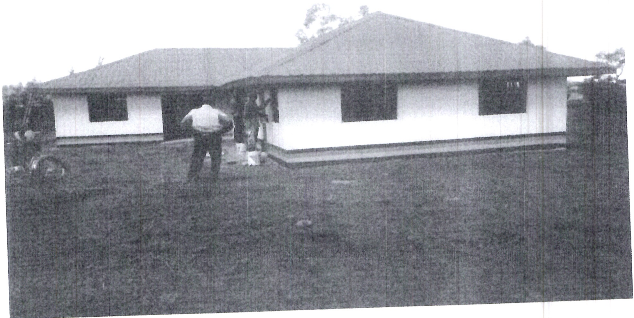
FIG1.2: Construction to completion of Ratanga Police Post in Ndhiwa financial year 2017-2018.
