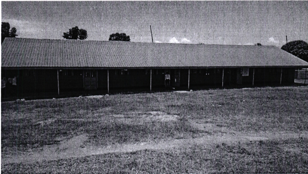
Pic 1: Kombewa MTC Four classrooms
