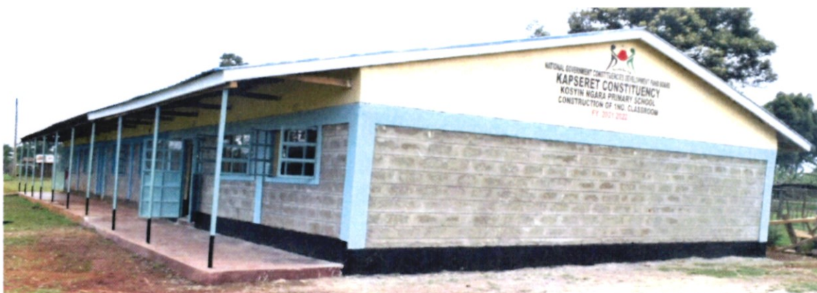
Kosyin Ngara primary school 3 classrooms
