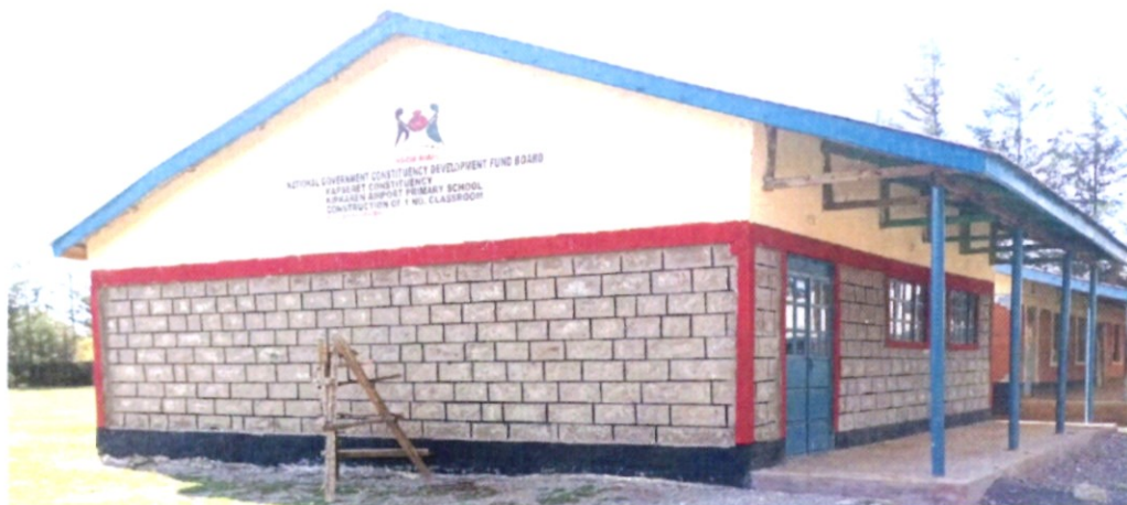
Kipkaren Airport Primary School 1 classroom
