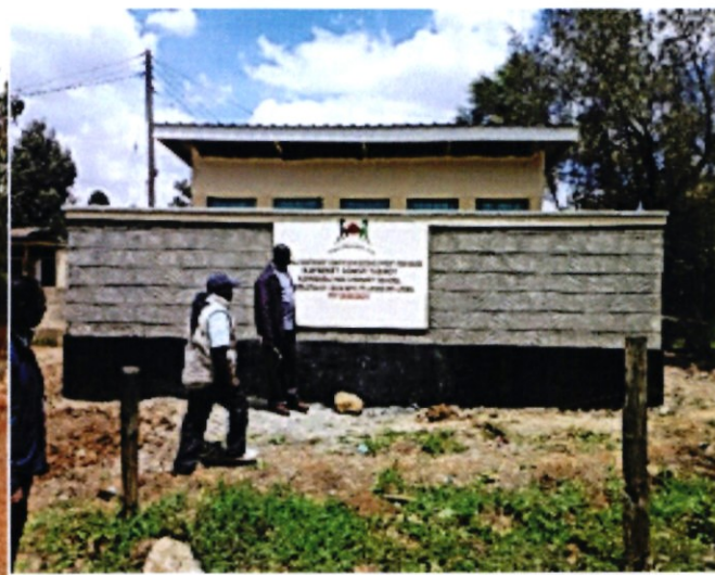
Kapkenduywo Primary School,5 Door boys latrine
