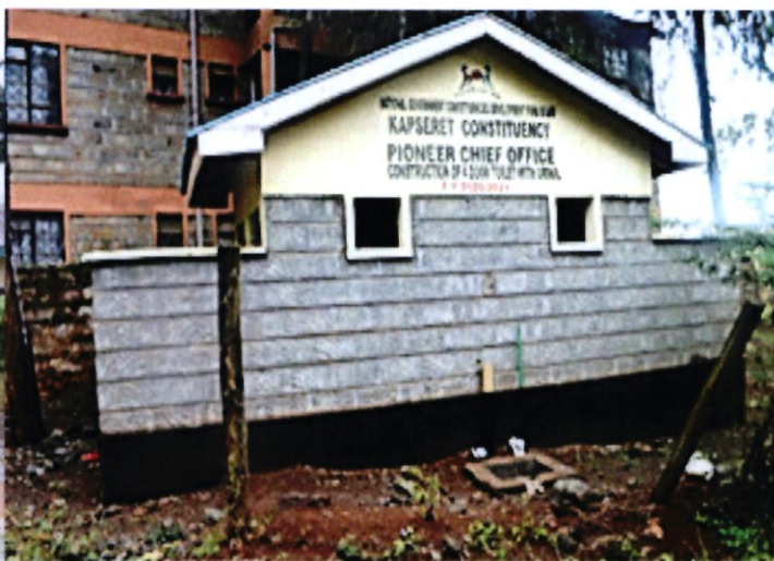
Pioneer Chiefs 4 door Toilets with Urinal
