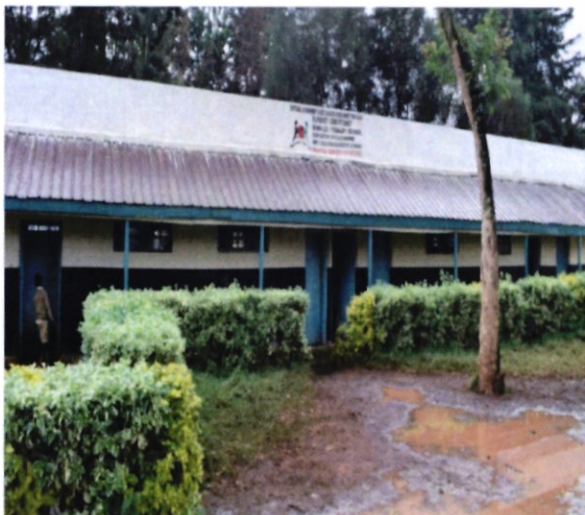
Kimalel Primary School Ablution Blook 21 door Renovations
